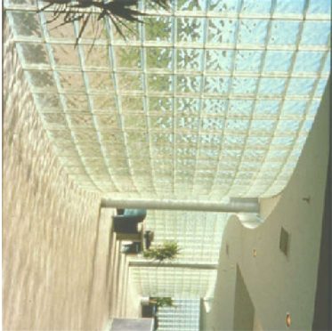
Example Images: Office walls to partially constructed from glass blocks to allow natural light to pass through
