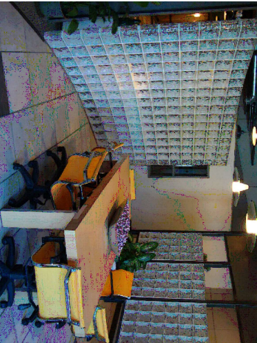
Example Images: Office walls to partially constructed from glass blocks to allow natural light to pass through
