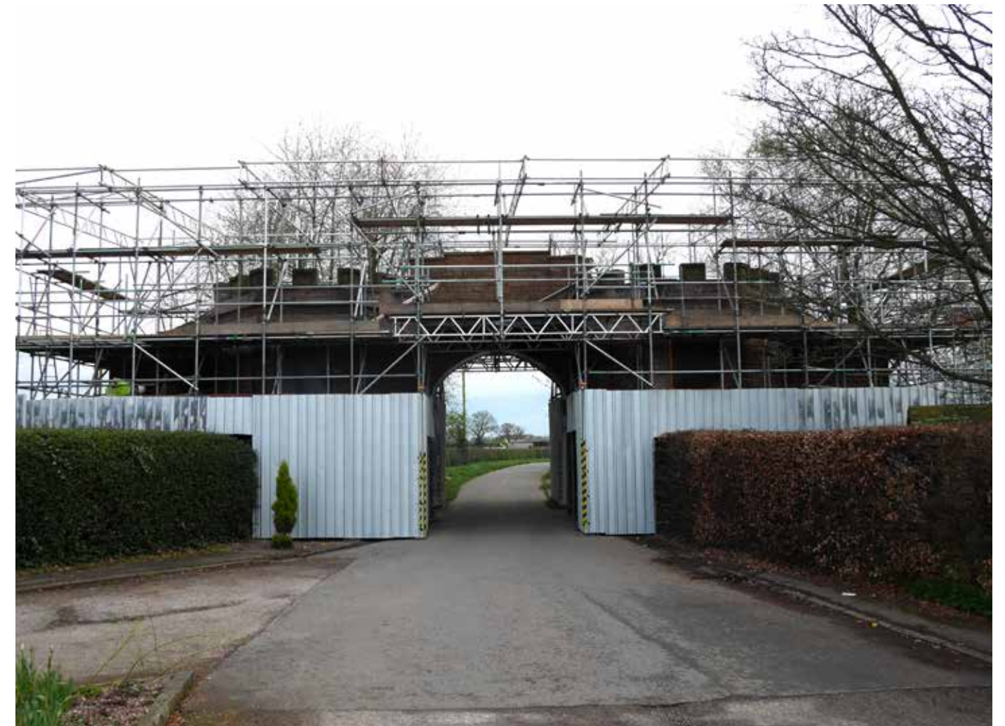
Restoration to a private residence, including a full repoint and masonry repairs, full re-roofing scheme, and overhaul to windows, doors, and cast iron rain water goods
