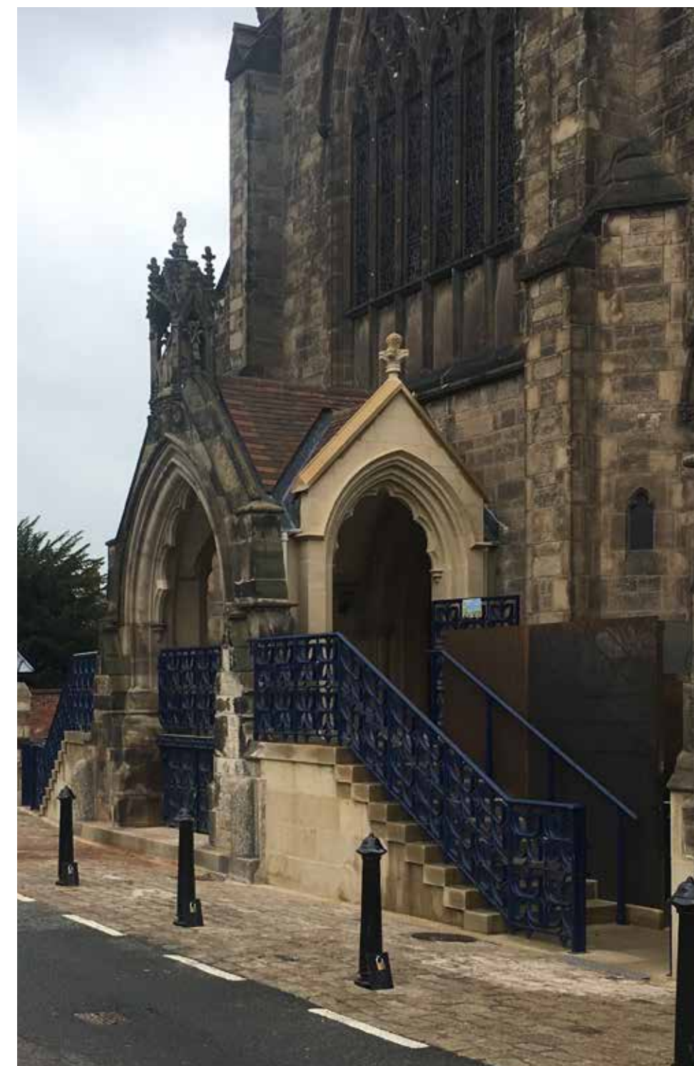
New disabled access entrance to the Cathedral, incorporating steps, access lift, ramp and four way pitched roof.
