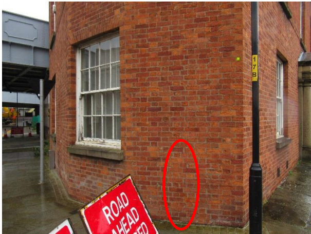
Western façade of the Station Masters House
