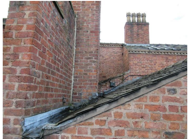
Roof transition between the Station Building and the Station Masters House
