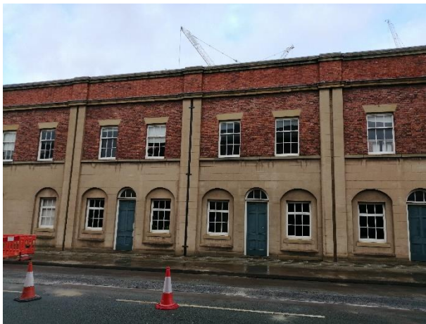
South façade as viewed from Liverpool Road
