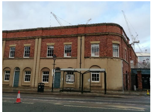
Eastern end of south façade
