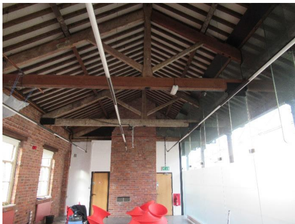
King post trusses at first floor over the rebuilt section of the building
