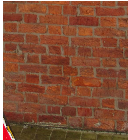
Cracking in masonry to western façade
