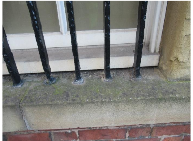
Railings embedded in the stone sill
