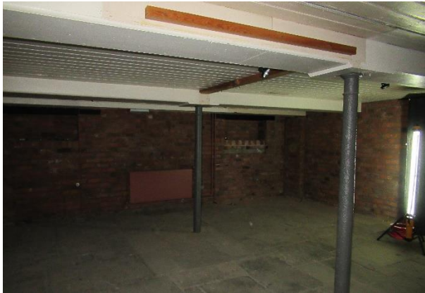
Downstand beams and cast iron columns at basement level
