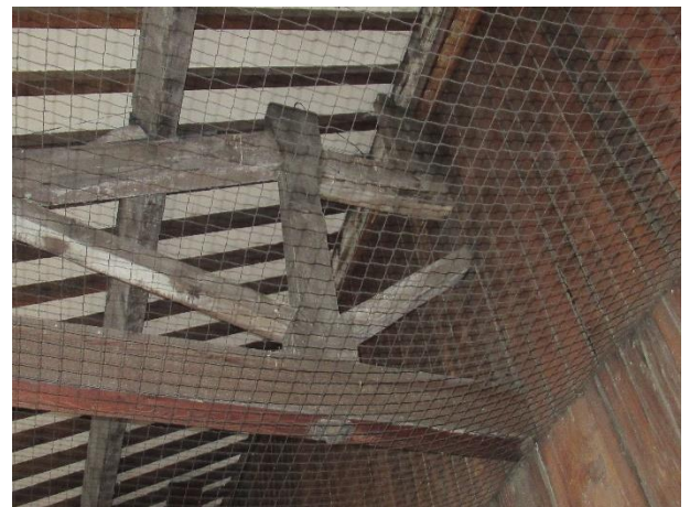
Queen post trusses to the western (not rebuilt) end of the platform
