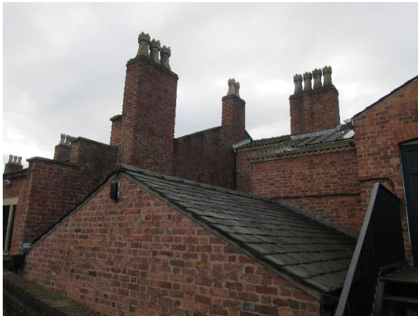
Station Master House roof construction
