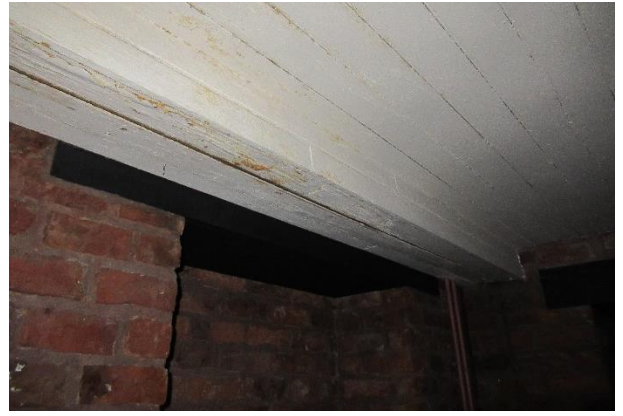
Recess in basement wall
