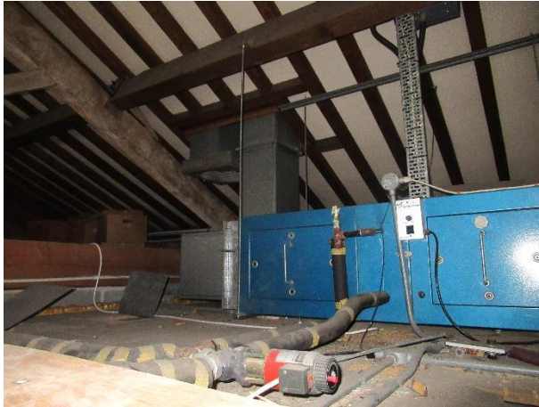
Ventilation over the waiting rooms at the western end of the Station Building
