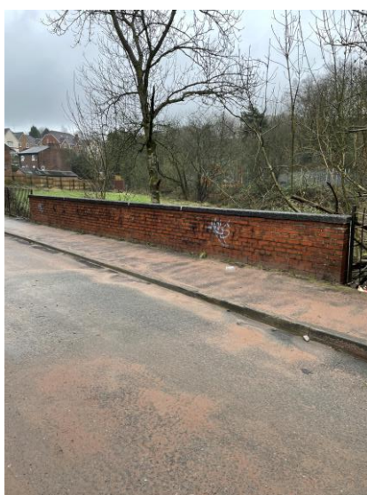
Figure 6 Gore Brook Bridge Parapet (Easterly Side)
