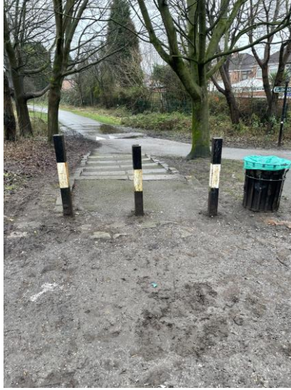
Figure 13 Steps at Stockport Branch Canal Northerly End
