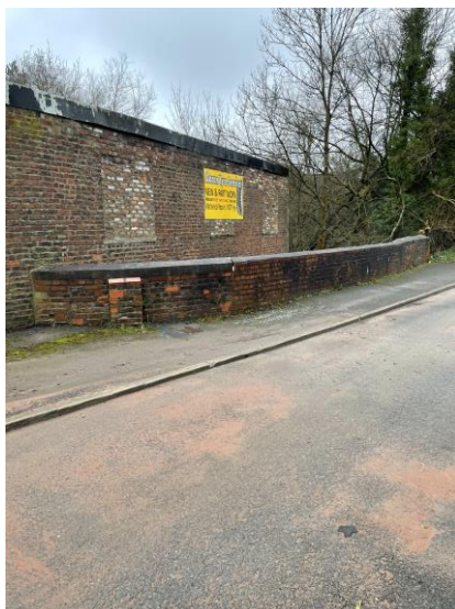
Figure 5 Gore Brook Bridge Parapet (Westerly Side)
