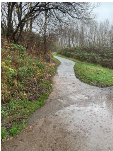
Figure 11 Ramp near bridge Number 6
