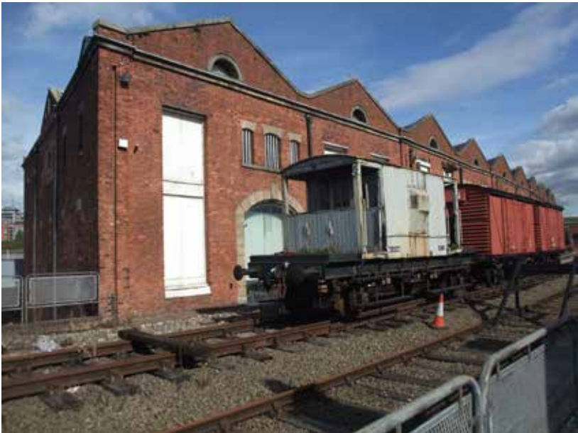
The south elevation looking east from the station platform
