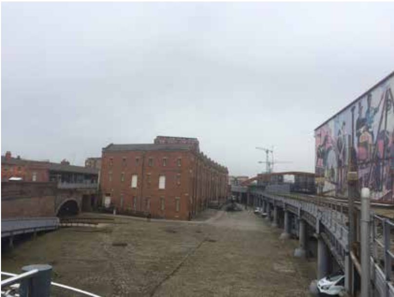
Looking west from the upper yard
