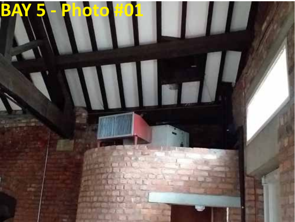
Photo #01 shows the existing hatch in relation to the purlin, and the existing M&E equipment to be removed.
