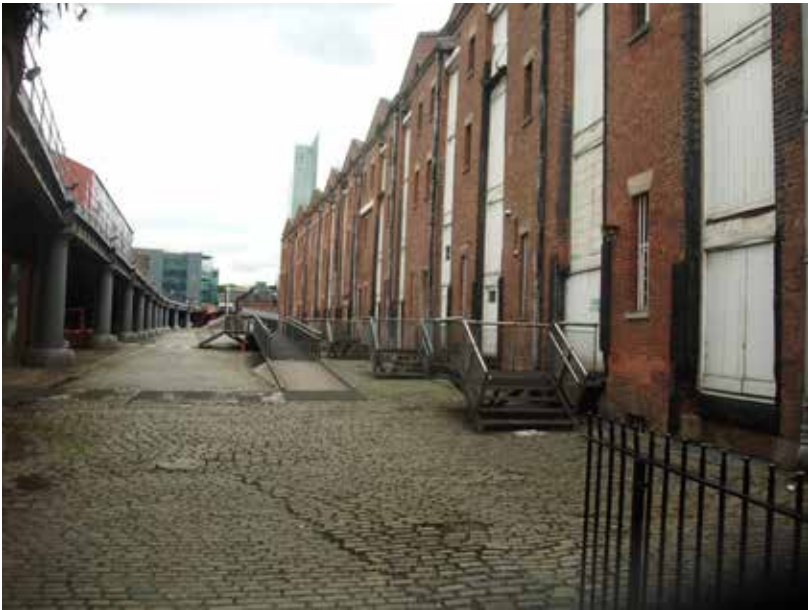
The north elevation looking east from the lower yard
