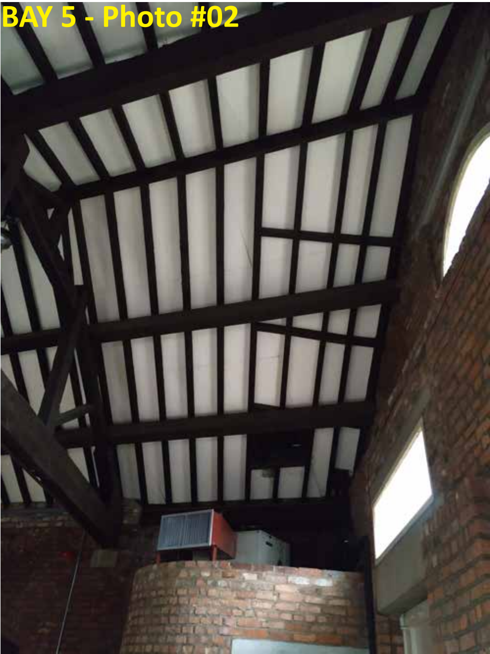
Photo #02 shows the existing rafter and purlin layout.
