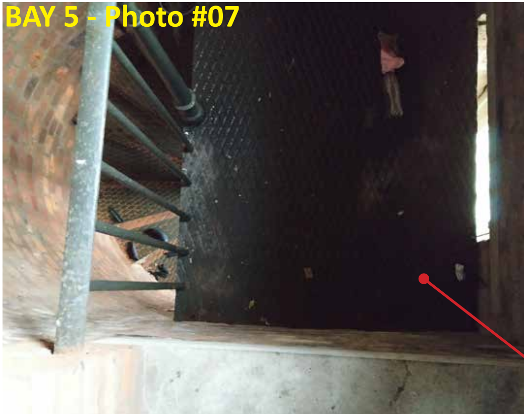
Photo #07 shows a detail of the existing central column rising to form the end of the balustrade.
