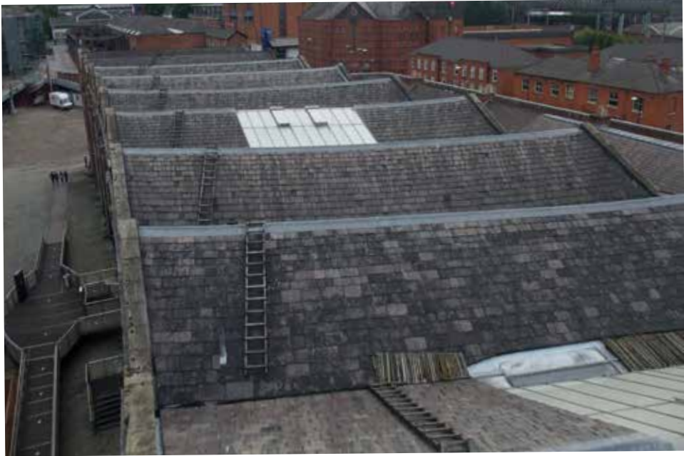
View of the roof looking East
