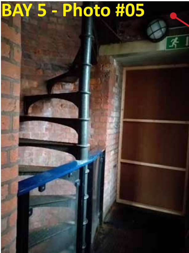
Photo #05 shows the existing spiral stair on the first floor rising to the existing lower platform on the second floor.
