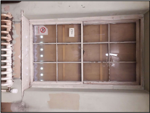
P22 - Internal View of Break Out Area A1/18 Security Boarding to external window WF No.5 to be removed & mesh grille fitted to match adjacent existing windows.
