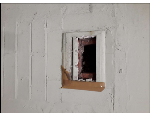
P22 - Internal View of Break Out Area A1/18 Security Boarding to external window WF No.5 to be removed & mesh grille fitted to match adjacent existing windows.
