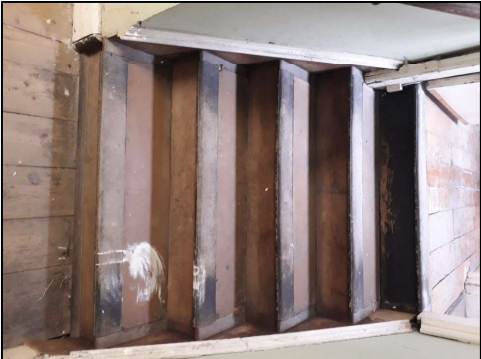
P23 - View of Break Out Area A1/18 Linoleum to treads of steps to be removed and replaced with new covering and nosings.
