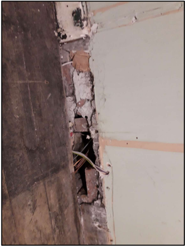
P19 - View of Break Out Area A1/18 To infill holes in base of wall where services penetrate and to fit new section of timber skirting, section and profile to match existing.
