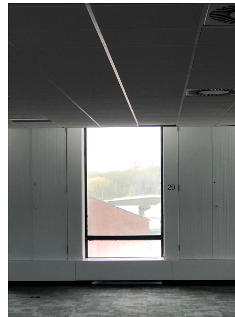
Existing suspended ceiling
