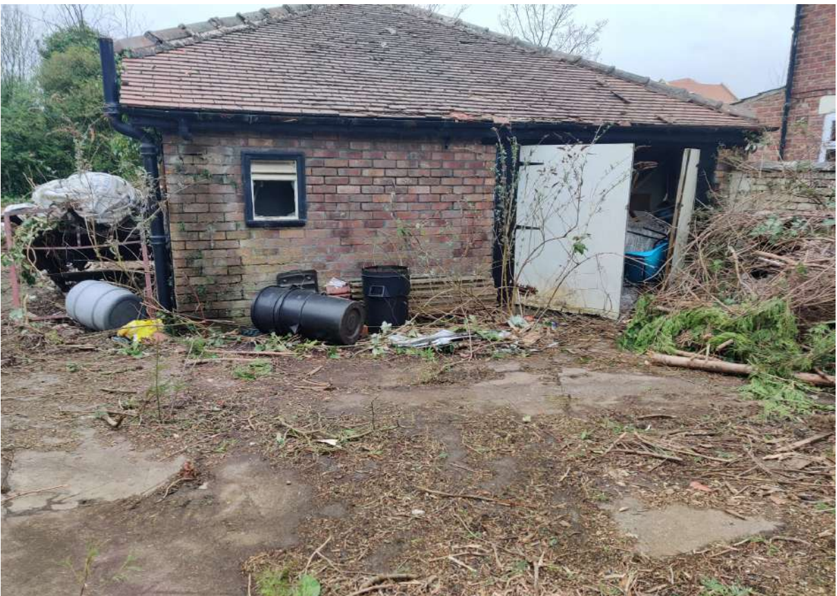
Photograph 4: View of the outbuilding in the west of the Site
