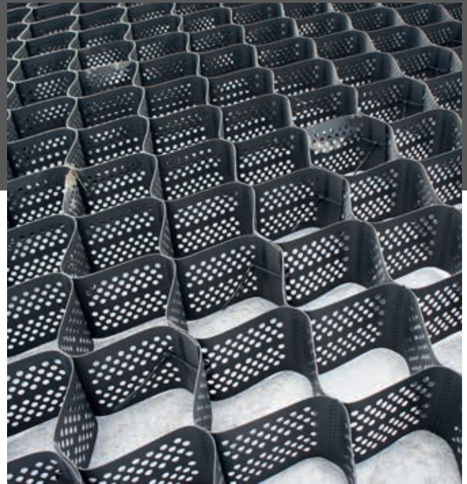
ProtectaWeb™ TRP System being pegged out
