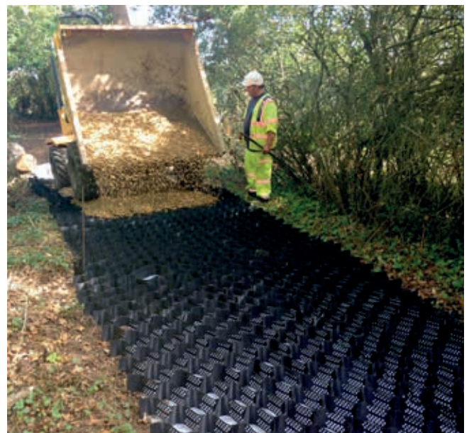
ProtectaWeb™ TRP System being infilled with stone
