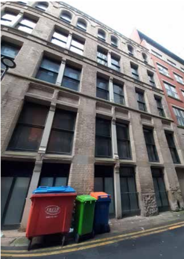
3.19c Back George Street elevation, plainer rear bays
