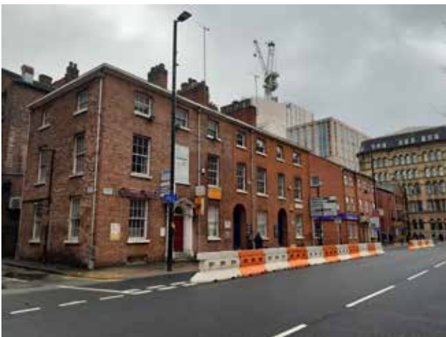
3.10 Georgian townhouses at 87-91 Princess Street
