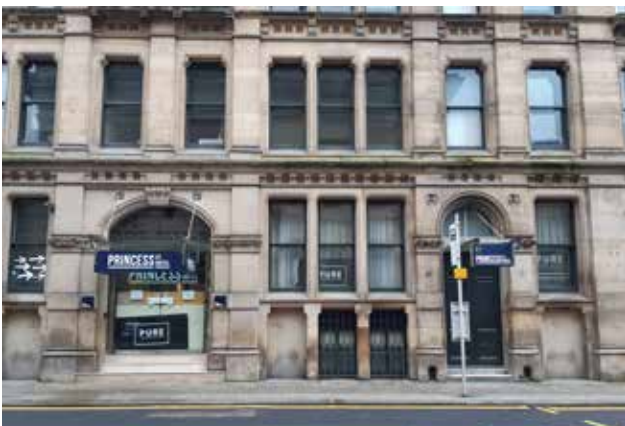
3.17a Raised ground floor entrances, modern glazing with metal work above to central opening and timber panelled doors to right-hand side
