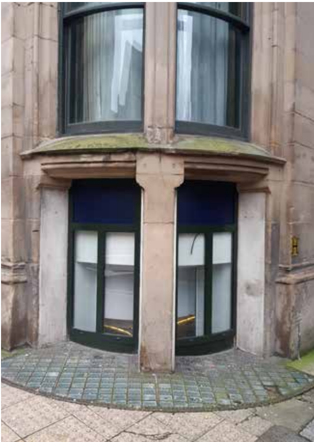
3.18a Basement lightwell infilled with pavement lights
