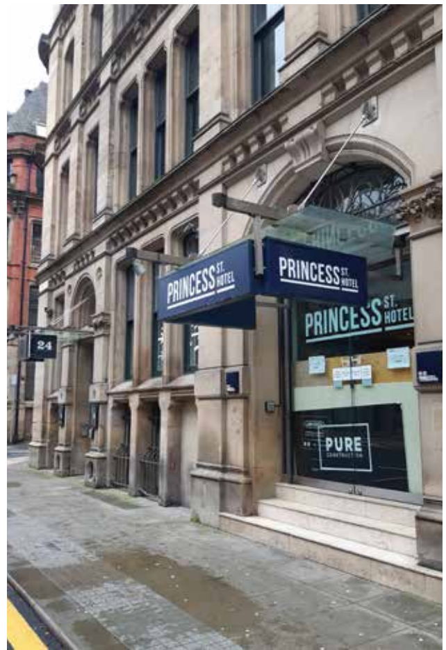
3.17c Detracting projecting canopies and signage
