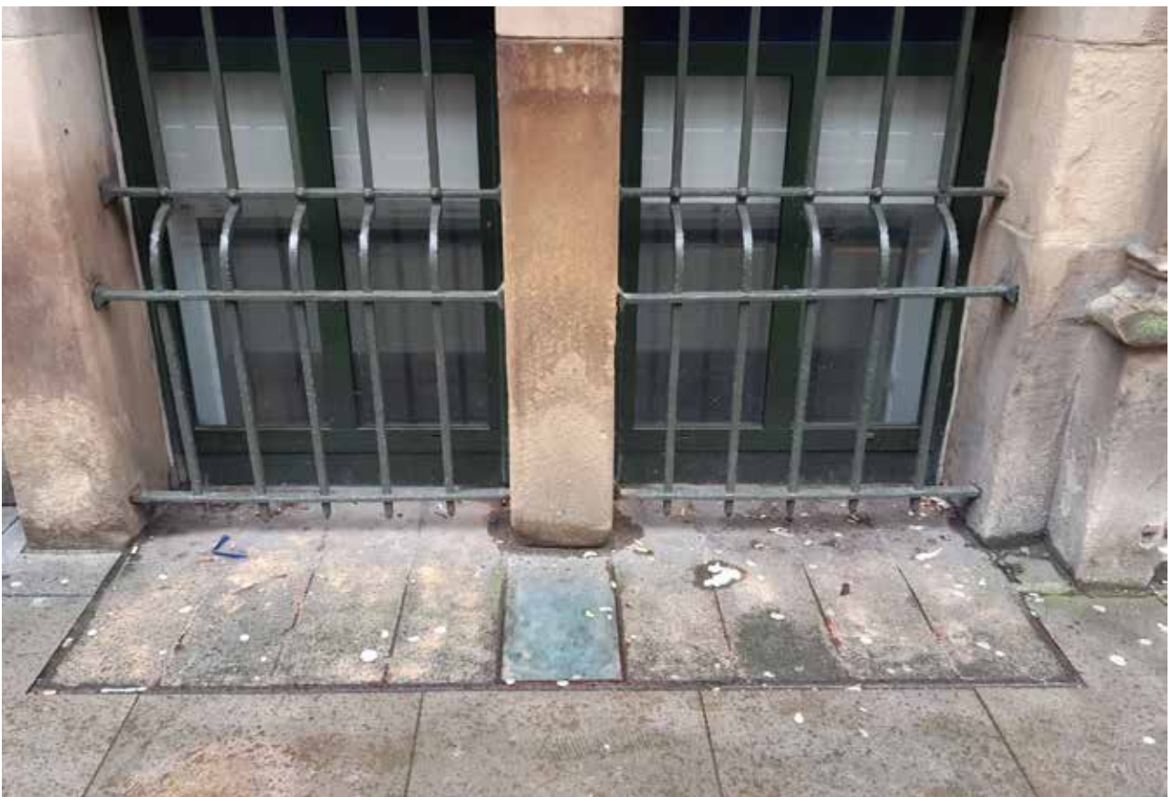
3.18b Basement lightwell infilled and later covered, railings to basement casements
