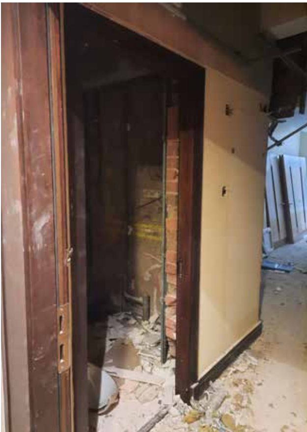
3.32a Original external wall now internalised
