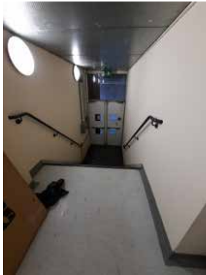
3.22c Rear modern staircase exiting on to Back George Street and serving all floors
