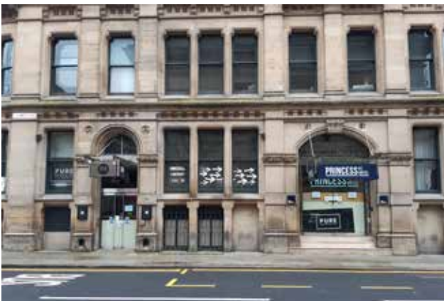
3.17b Lowered ground floor entrances to left-hand side to provide level access with modern glazing
