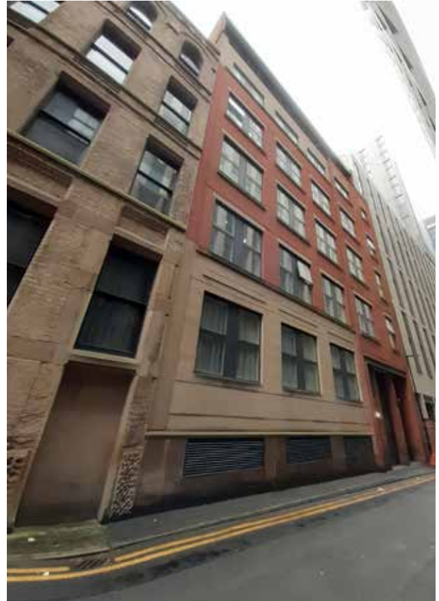
3.20d Modern infill development in place of 53 Back George Street
