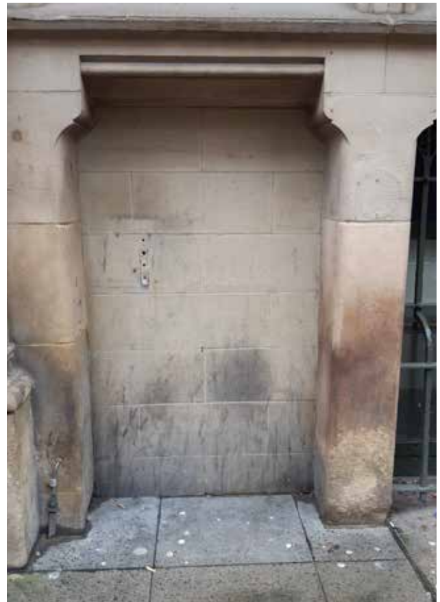
3.18c Basement opening infilled with blockwork and pavement extended over lightwell
