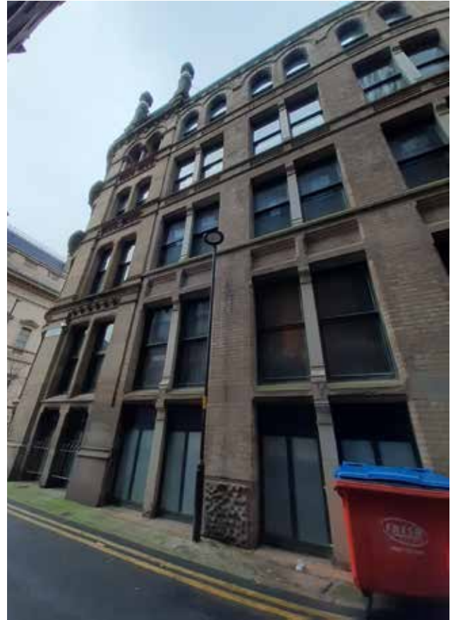
3.19b Back George Street elevation, return two bays continuing principal facade detailing
