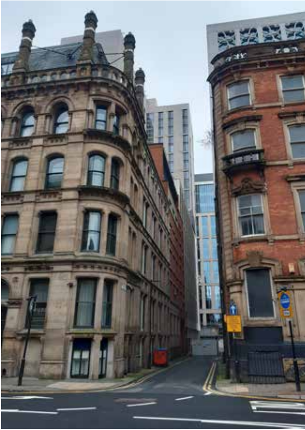
3.14 View down Back George Street with contemporary development on and behind St Peter's Square behind
