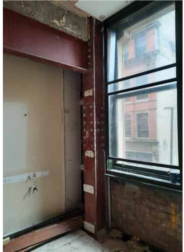
3.29b Opening up works at first floor revealing modern structure
