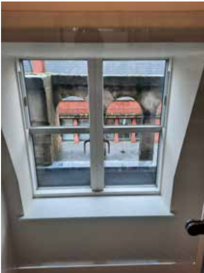
3.21b Casement windows at 4 th floor behind parapet
