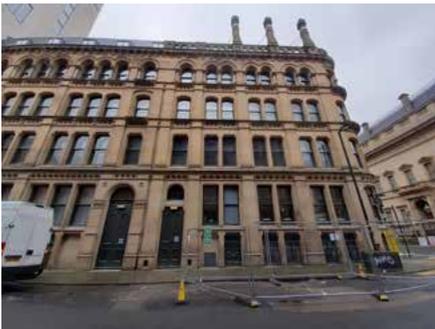
3.20b George Street elevation, paired window bays and secondary entrance to Princess Street building
