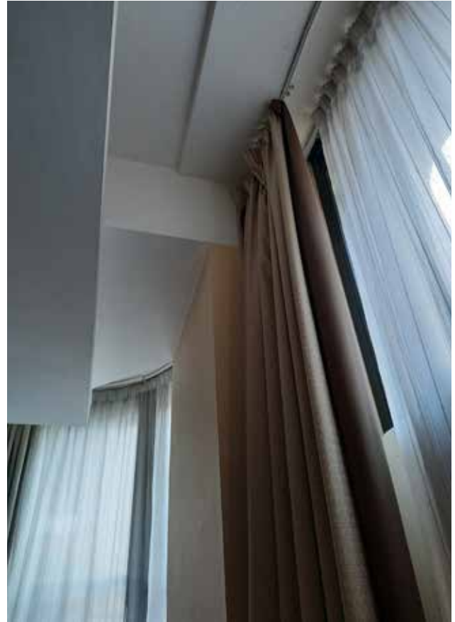
3.25c Awkward relationship between lowered ceilings and window openings
