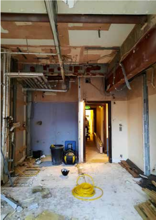
3.29a Opening up works at first floor revealing modern structure
