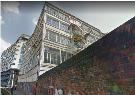
Pic 4 shows the view looking east from the Rochdale canal towpath along the northern perimeter of Barclay House.
