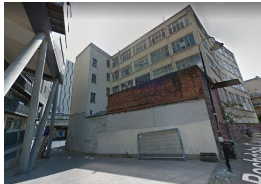
Pic 5 shows the view looking west from the Rochdale Canal towpath at the eastern perimeter of Barclay House.
