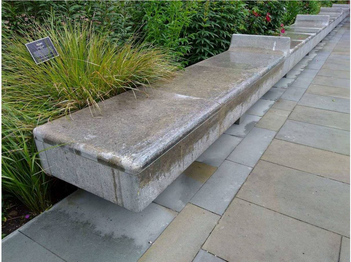
Photo 9. Close up damage to bench
