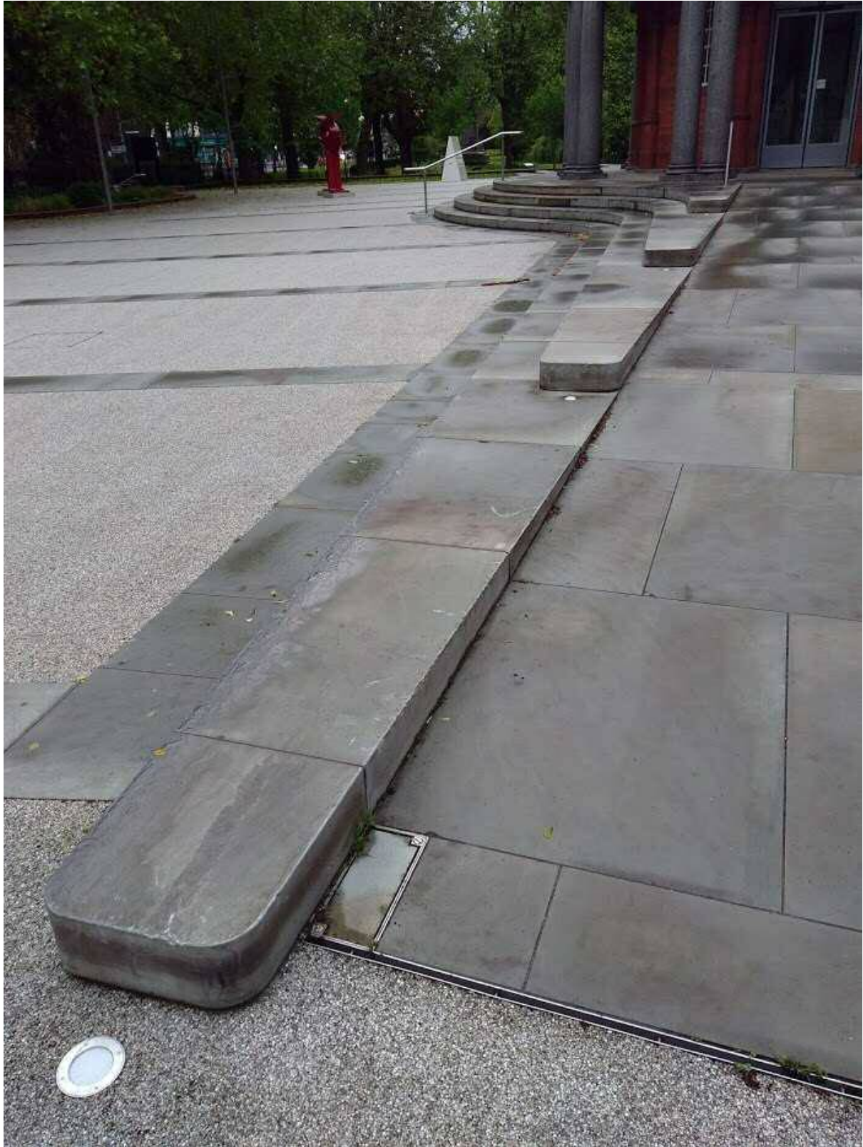
Photo 2. View of steps to side of access ramp
