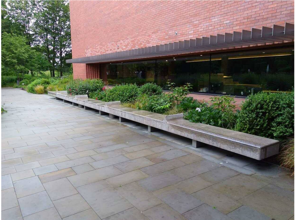
Photo 7. Benches - Viewed from rear entrance
