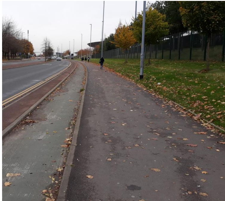
Photo 4: Footway on Alan Turing Way
