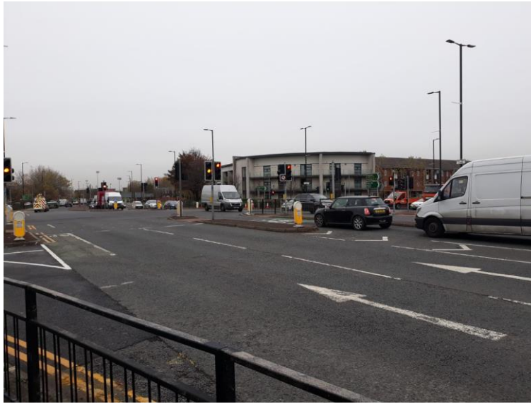
Photo 3: Alan Turing Way/A635 Signalised Junction
