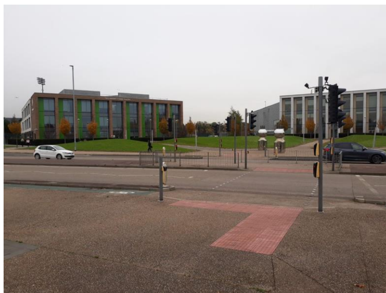
Photo 5: Staggered Toucan Crossing on Alan Turing Way
