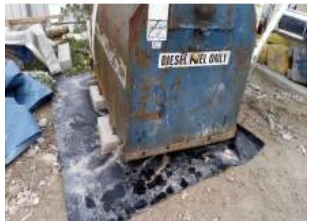
Figure 2.5: Diesel storage tank adjacent to the mortar silos in the northwest of the site.
