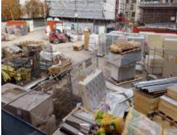
Figure 2.3: General view across site, looking north from cabins in southwest corner.
