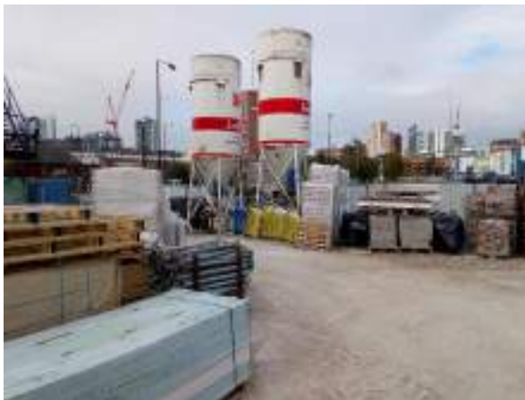
Figure 2.5: Looking towards the mortar silos in the northwest of the site.
