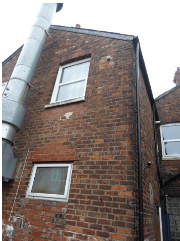
Photograph 3. Rear elevation of outrigger at high level.
