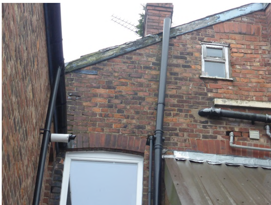
Photograph 5. Rear elevation at high level
