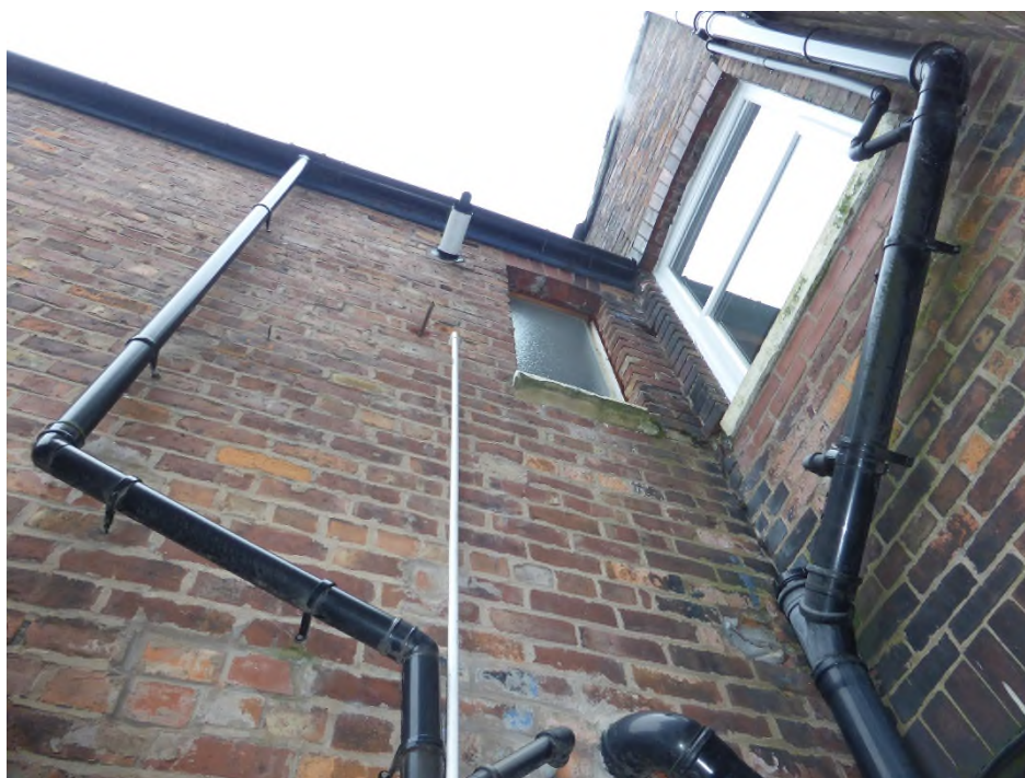
Photograph 6. Rear elevation at high level
