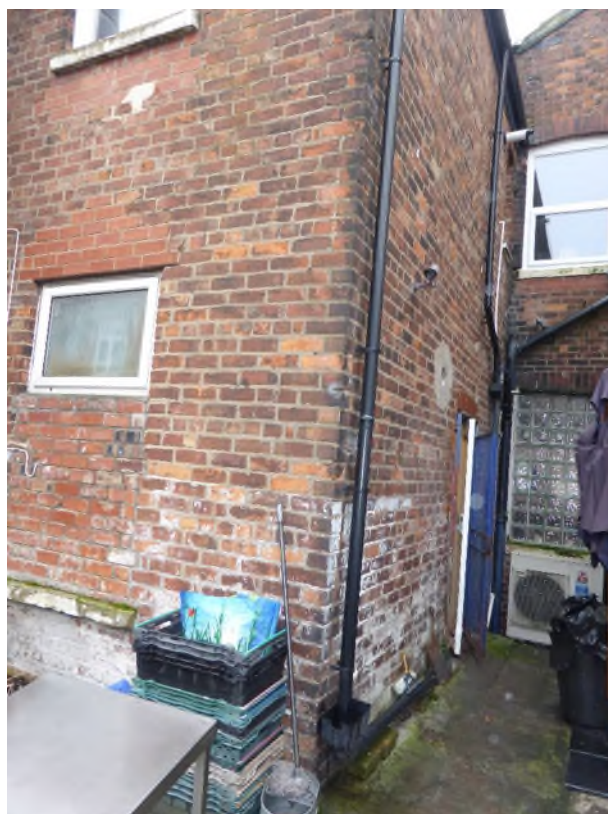
Photograph 4. Rear elevation at low level
