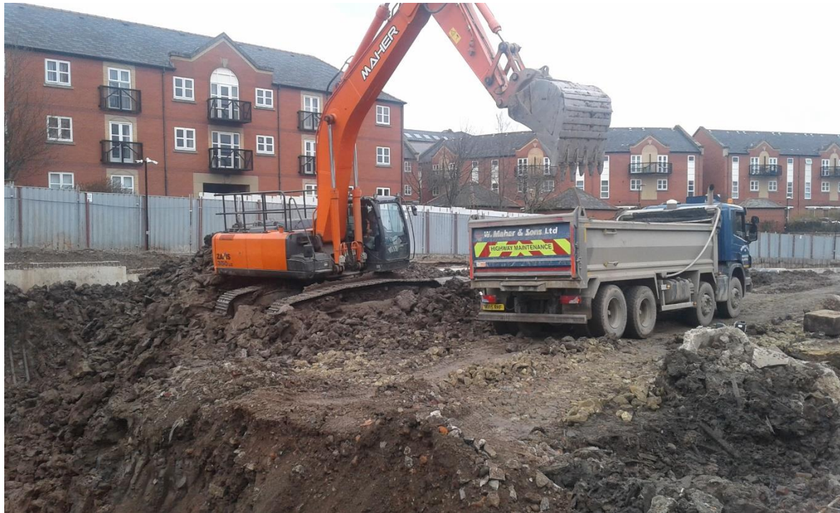
PLATE 1 – REMOVAL OF SOILS AS PART OF THE REDUCED LEVEL DIG
