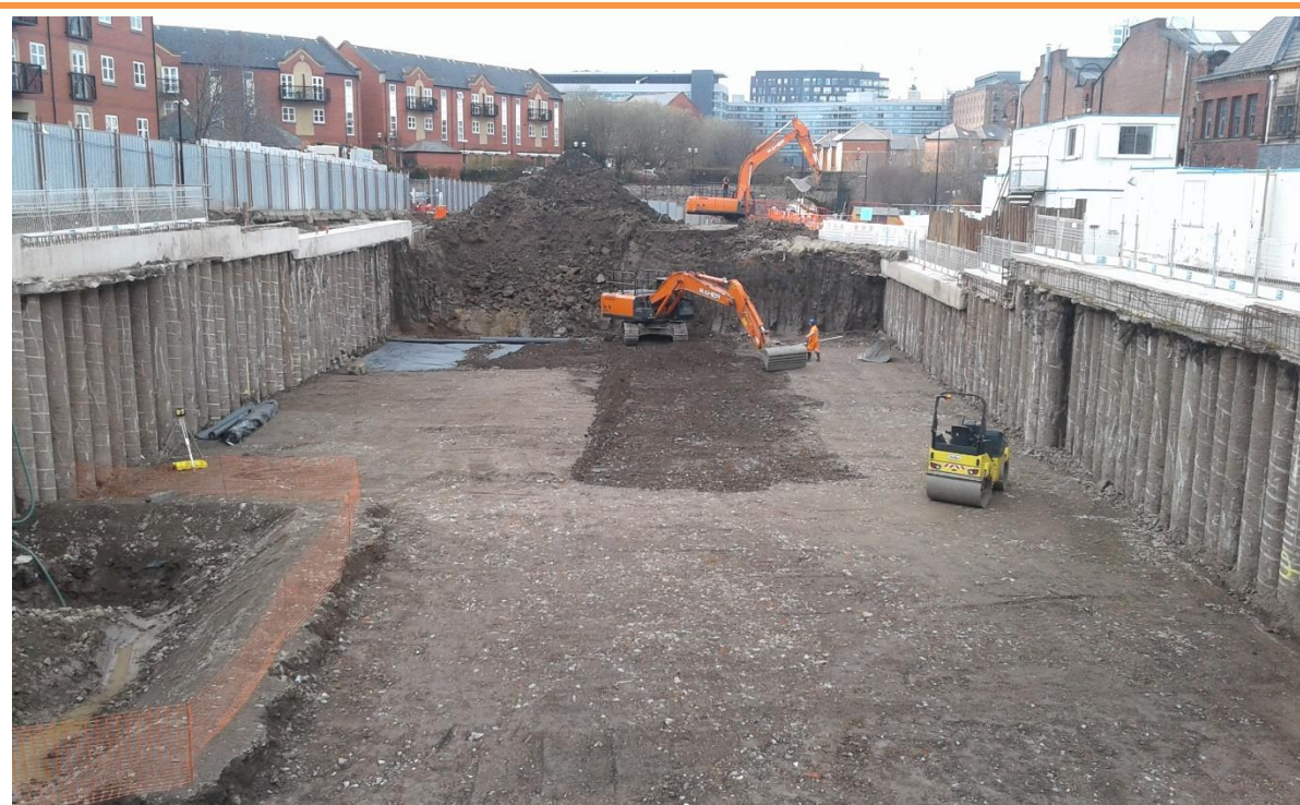
PLATE 3 – REMOVAL OF SOILS AND CONTINUED INSTALLATION OF PILE MAT
