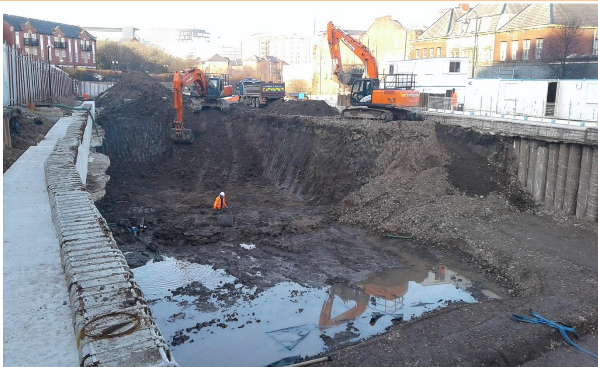
PLATE 2 – REMOVAL OF SOILS AND INSTALLATION OF PILE MAT
