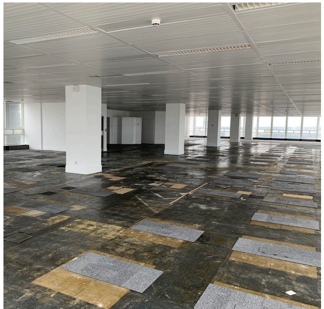
Level 15 (highlighting carpet, lino and paint on top of screed)
