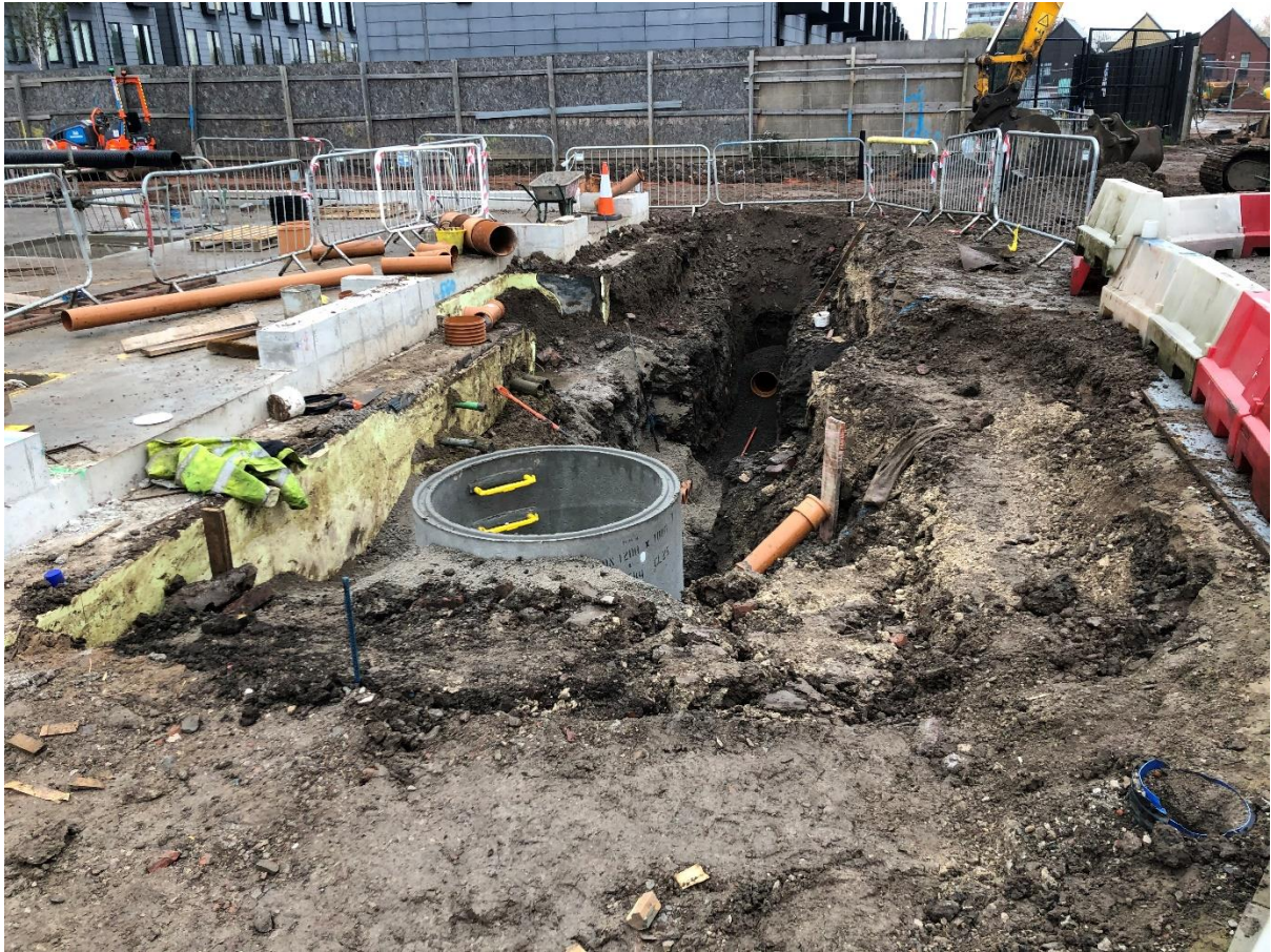
Figure 4 shows the construction of surface water manhole S13.
