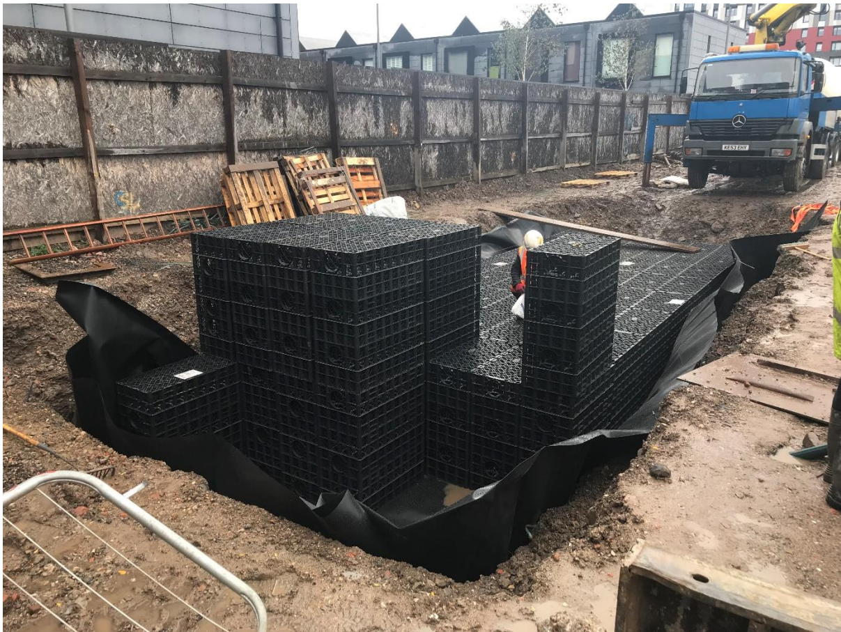
Figure 1 shows the installation of the surface water drainage cellular attenuation tank in the car park area in front of Mansion House.
