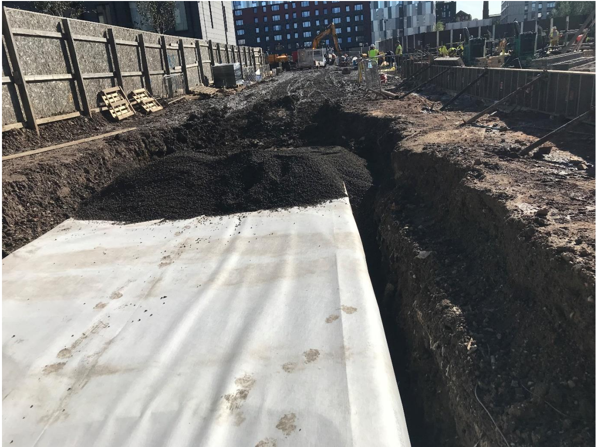
Figure 2 shows the membrane lining of the cellular attenuation tank prior to backfilling.
