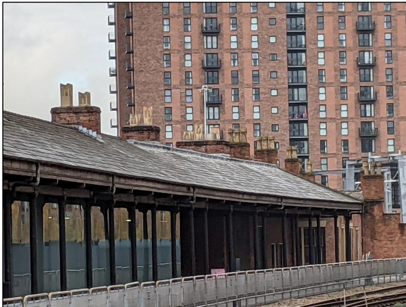
Photograph 3 showing the roof of the station building
