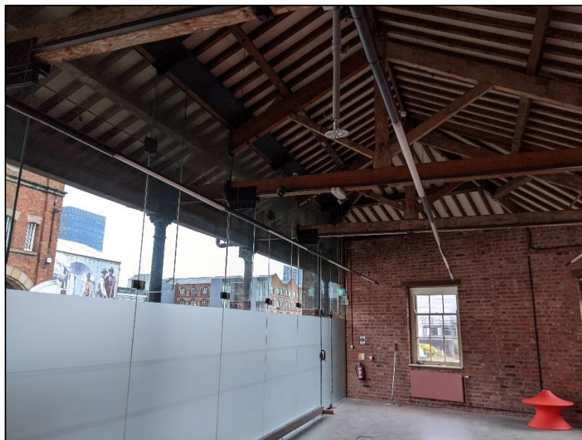
Photograph 6 showing the canopy of the former rail station
