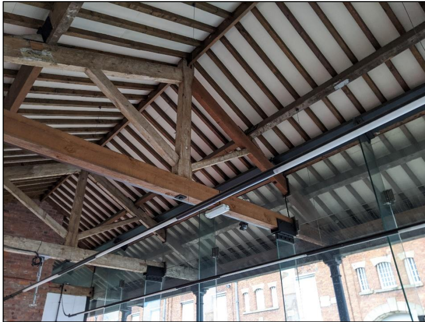
Photograph 5 showing the canopy of the former rail station
