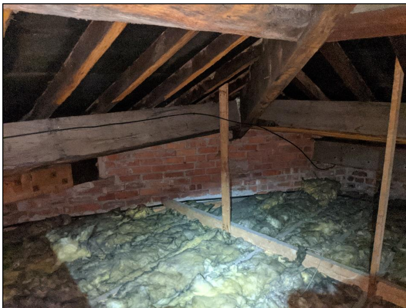
Photograph 8 showing the roof void of the Station Building
