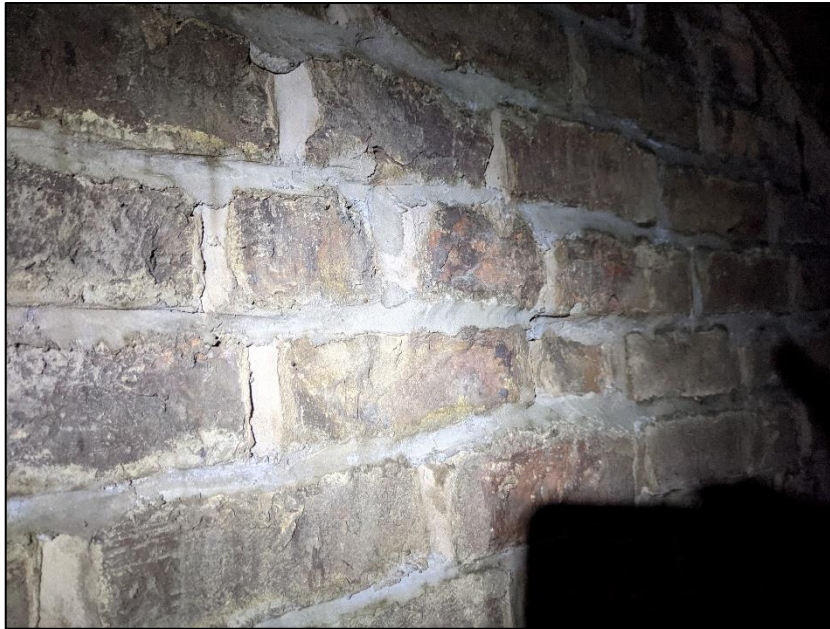
Photograph 9 showing the internal brickwork in the roof void
