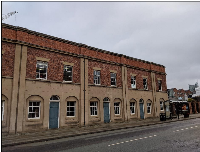
Photograph 1 showing the exterior of the station building
