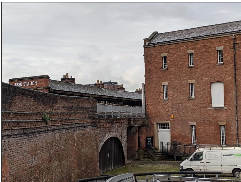
Photograph 4 showing the roof of the station building
