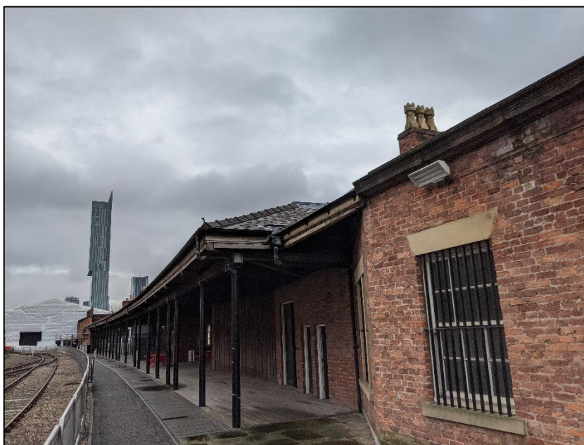
Photograph 2 showing the exterior of the station building
