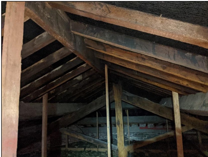
Photograph 7 showing the roof void of the Station Building
