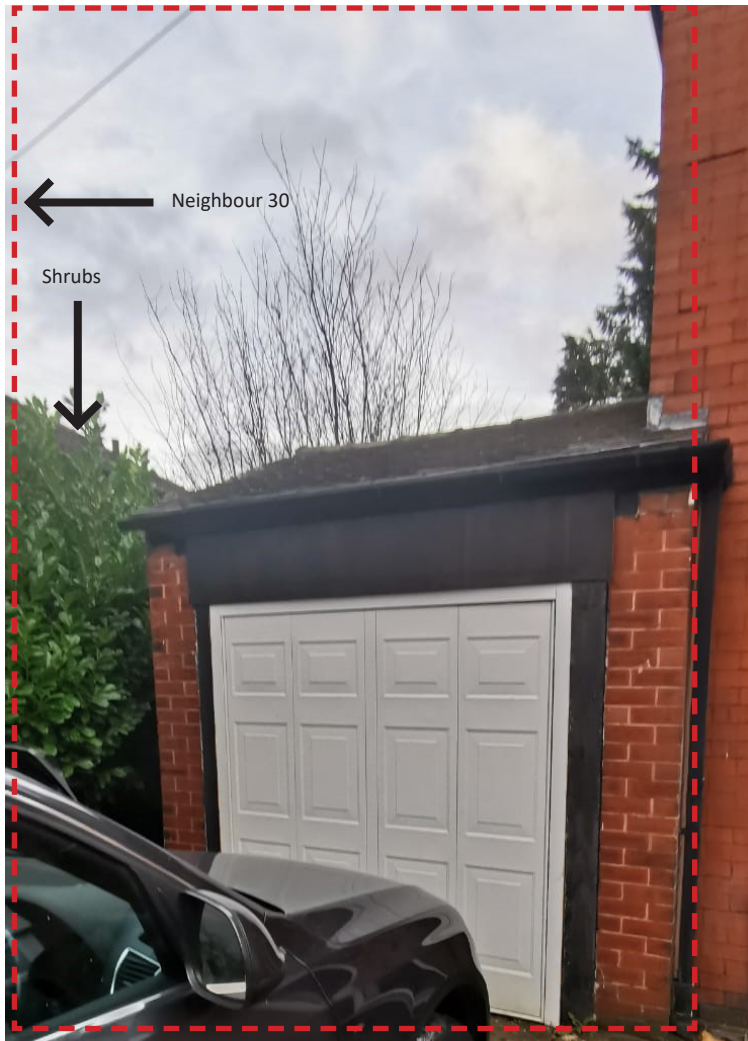
Fig 01 Existing Front View
