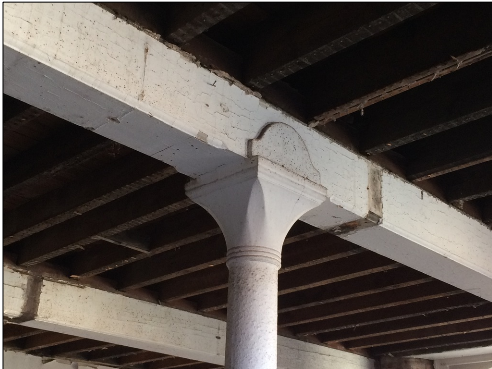
Plate 11: Typical cast iron column capital with clasp. Note chamfer and stop detail to timber joist.
