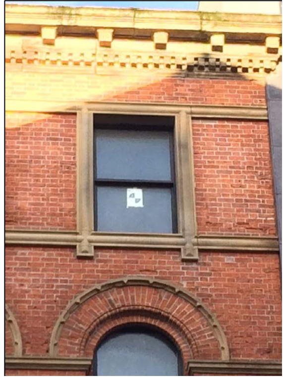
Detail 4: Third floor window arrangement, repeating the "dropped ear" detail of the first floor
