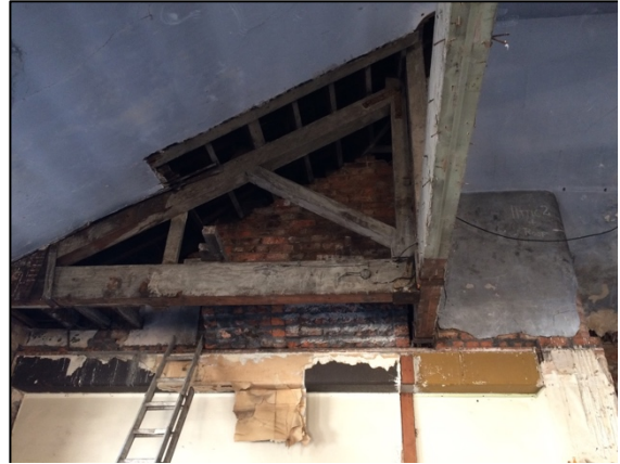
Detail 16: Corbelled chimney stack at high level attached to the stair enclosure of the third floor.
