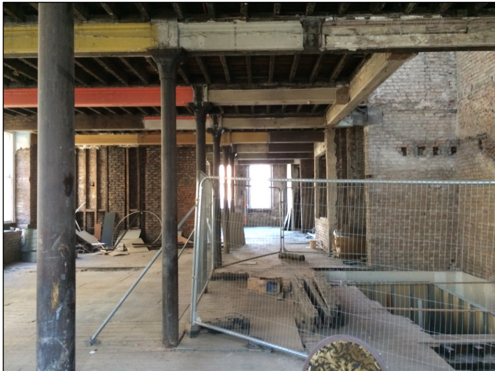
Plate 13: The first floor looking north with the original hoist void to the right
