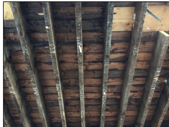
Detail 22: Typical ceiling arrangement at second floor level with marks for former lath and plaster visible where removed.
