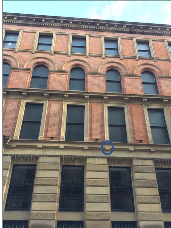
Detail 2: Typical section of the Southmill Street elevation showing dropped “ears” protruding into the ground floor from the first floor window surrounds (the “ears” circled in blue), a typical Mannerist detail.
