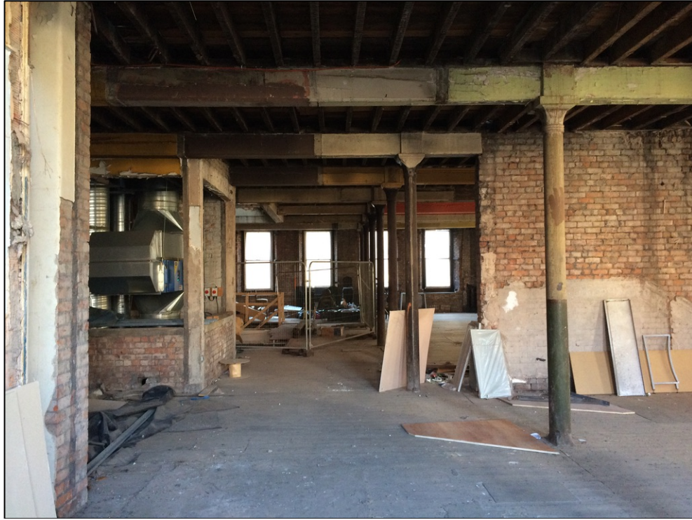
Plate 12: The first floor looking south with the staircase enclosure and secondary hoist to the left
