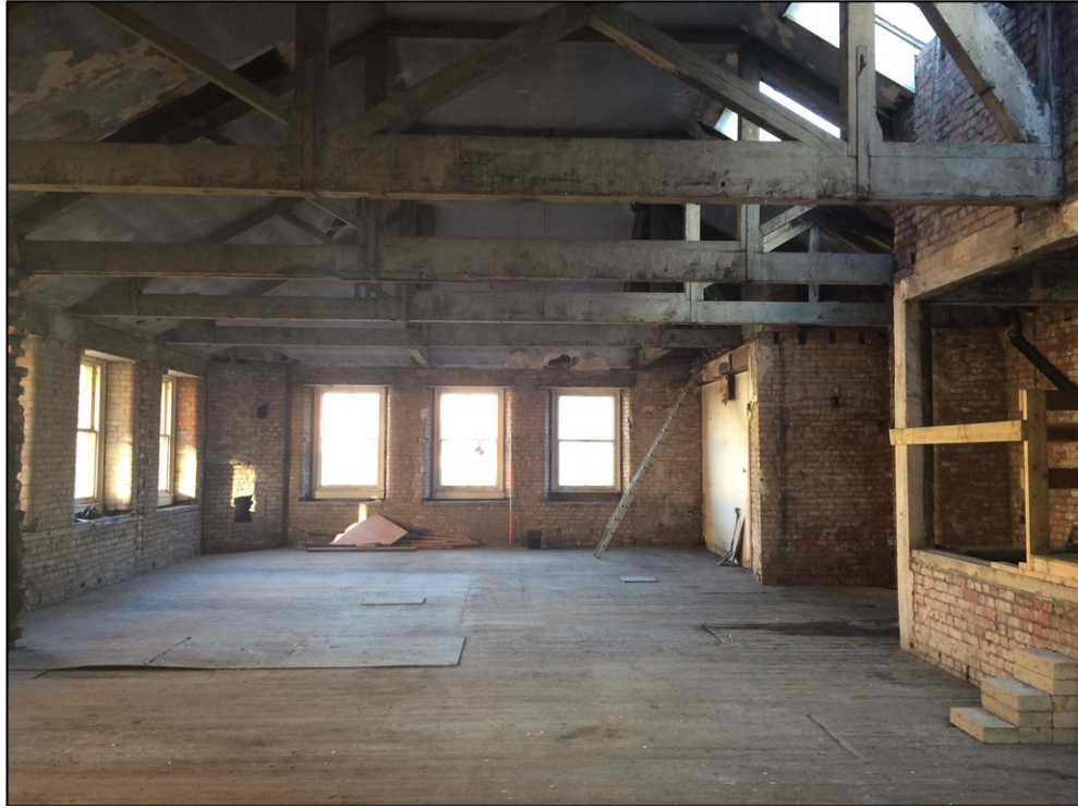
Plate 8: The third floor looking north with the secondary hoist and staircase enclosure to the right
