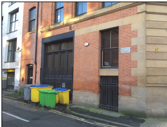
Detail 9: Location of former vehicle entrance to lower ground / basement floor, visible on Goad's map of c. 1885. Subsequently altered.
