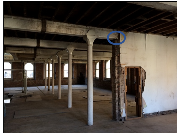
Detail 26: Truncated chamfer and stop detail (circled in blue) at second floor level confirming the brickwork partition to the right-hand side to be a later addition.
