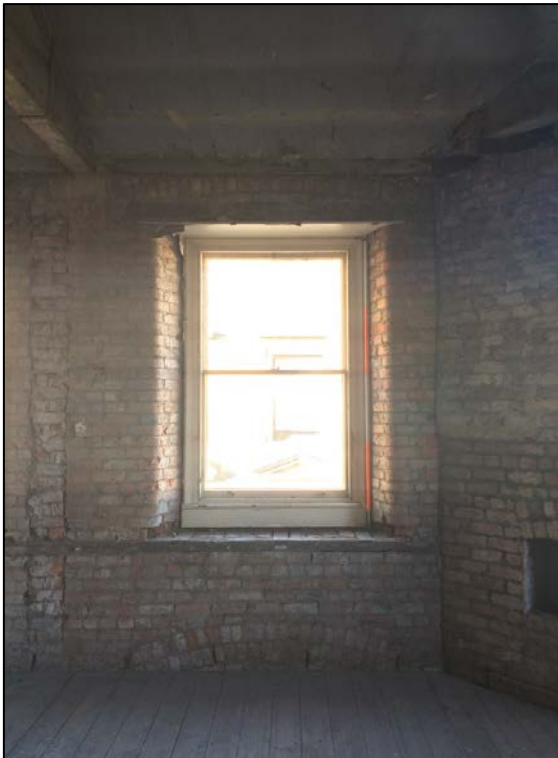
Detail 17: Typical one-over-one timber framed sliding sash window to third floor level.
