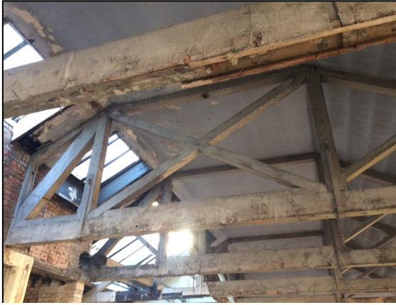
Detail 11: Strengthened roof truss (4 th from the north / Bootle Street). Possibly associated with additional loads from nearby hoist machinery.
