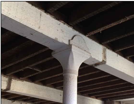
Detail 25: Typical cast iron column capital and clasp accepting timber joist above.
