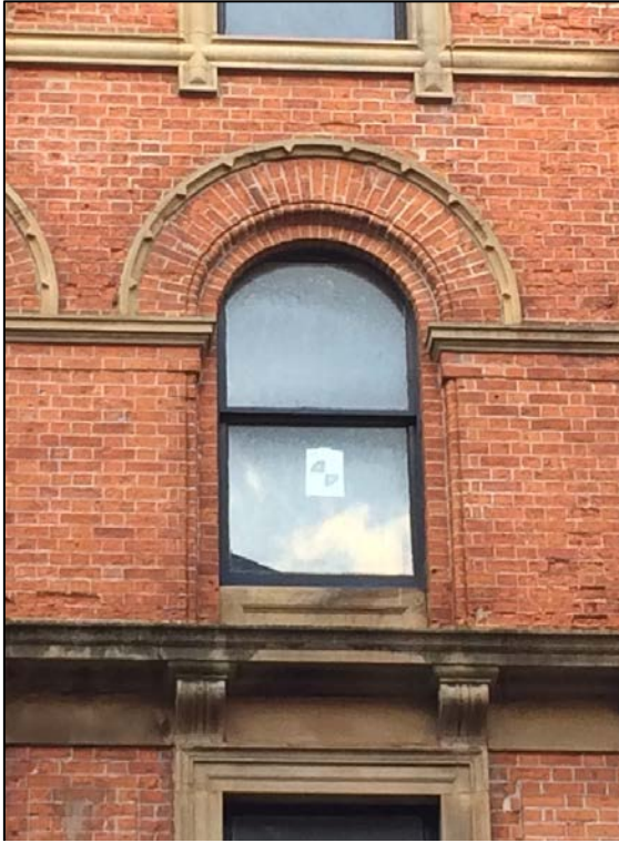
Detail 3: Second floor window arrangement with decorative stone moulding
