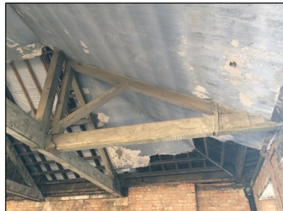
Detail 10: Truncated King Post truss section forming hip to south end of roof construction.
