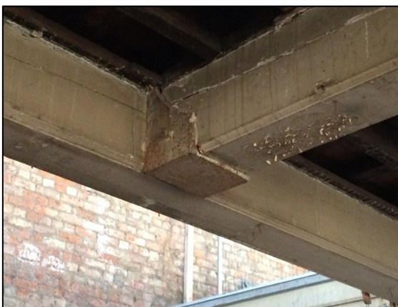
Detail 41: Original chamfer and stop details to timber joists enclosing hoist opening, confirming original arrangement of hoist in this location.
