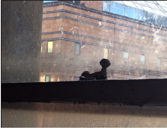
Detail 19: Typical original sash catch ironmongery detail to upper sash of windows.
