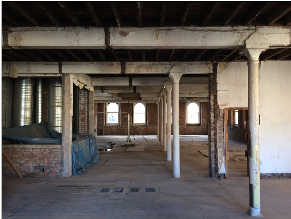
Plate 9: The second floor looking south with one of the offset cast iron columns to the right
