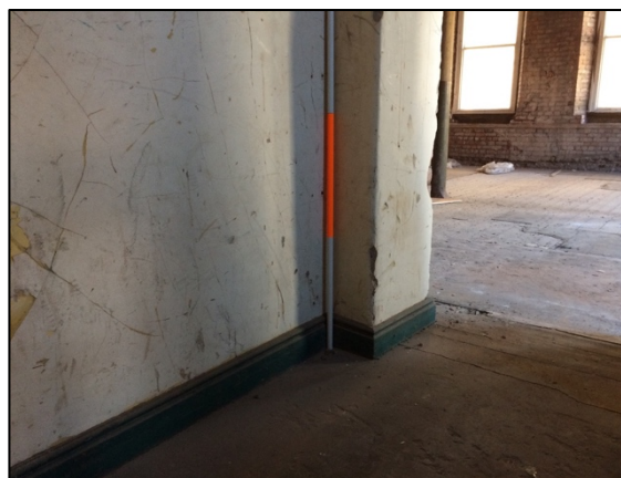
Detail 38: Fragmentary survival of timber skirting to first floor level of staircase enclosure.
