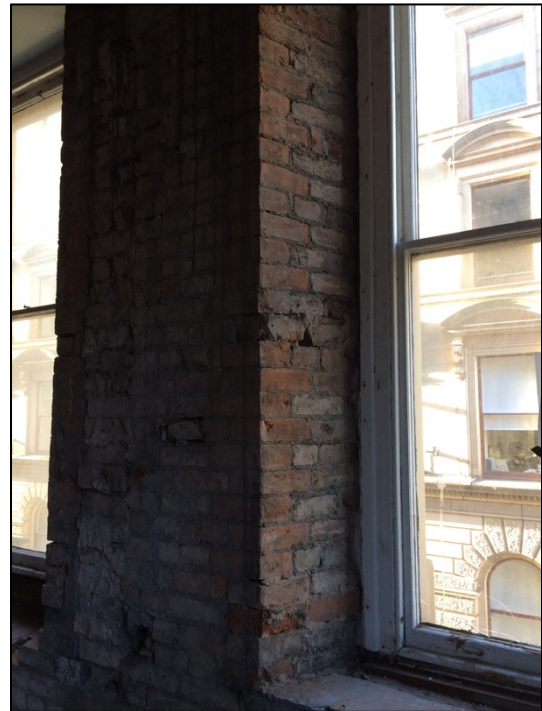
Detail 30: Chamfered window reveal at first floor.
