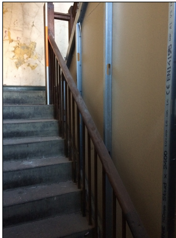
Detail 36: Surviving section of balusters to ground floor level of staircase.
