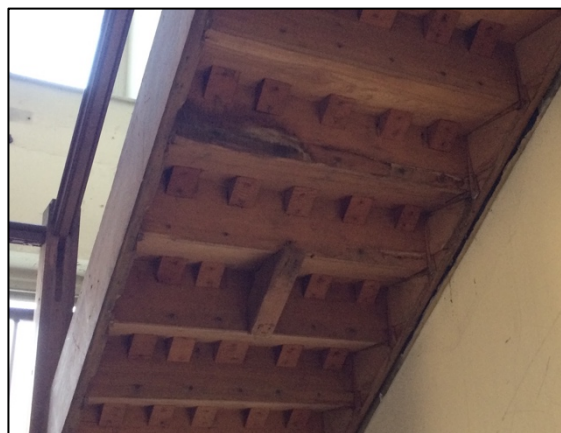
Detail 34: Typical view of the soffit of the c. 1950s timber replacement staircase showing the very high quality of construction to the treads and risers.
