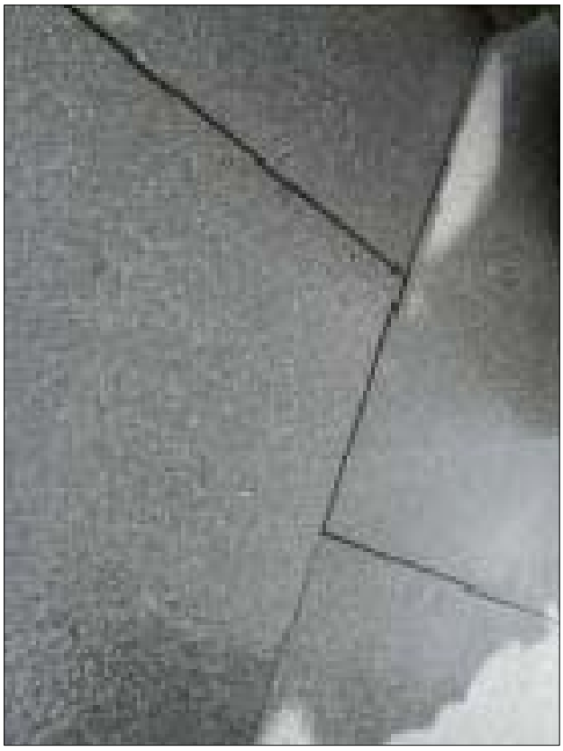
Resin bonded gravel with natural stone trim
