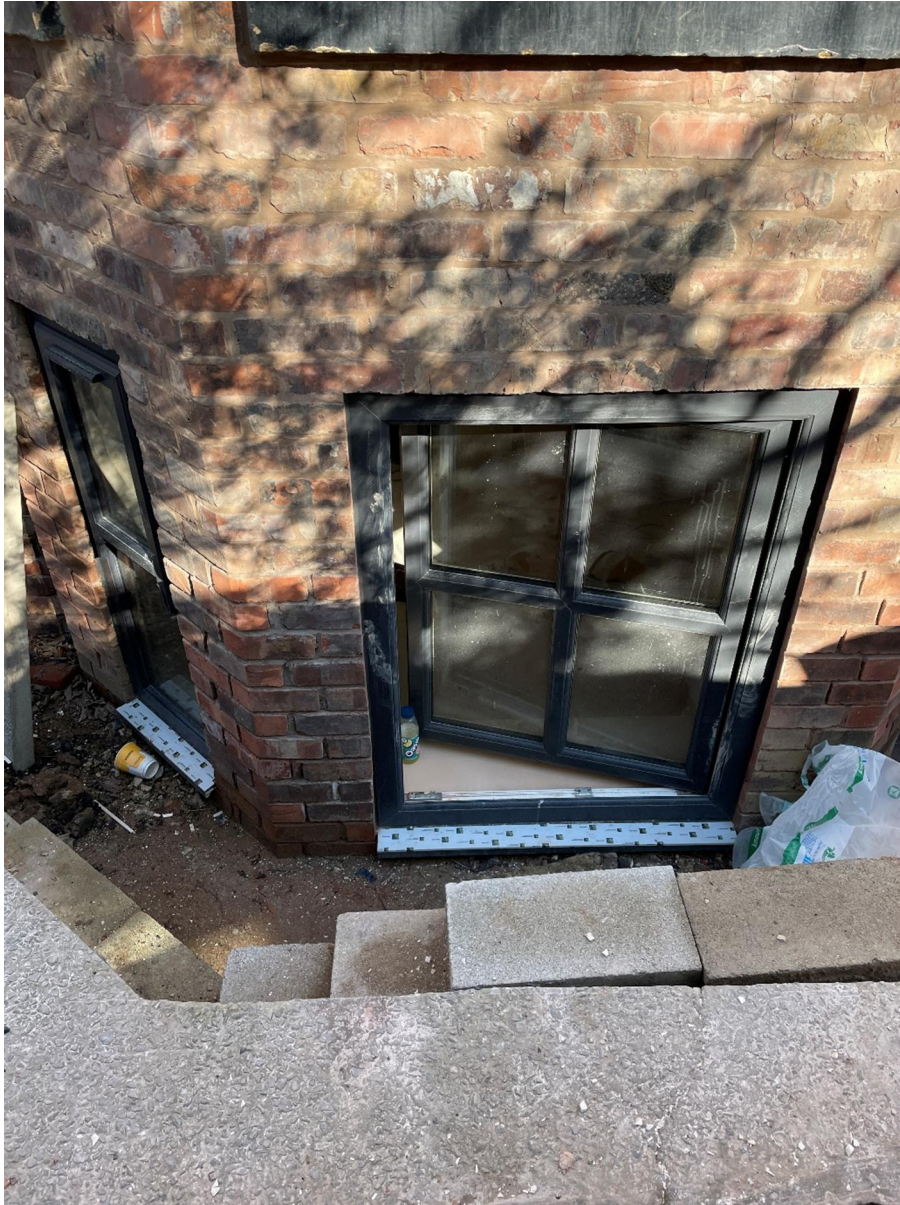
View on side lightwell bay
