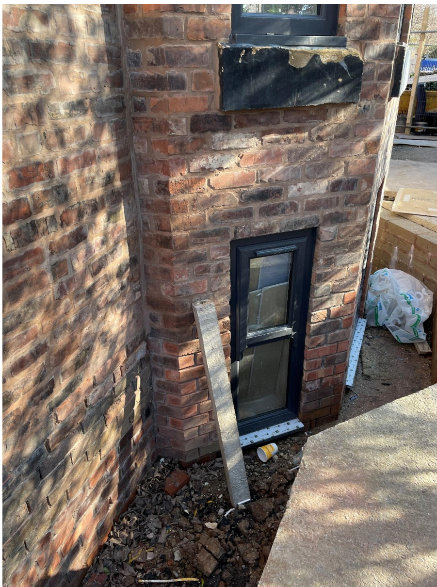
View of side lightwell from rear
