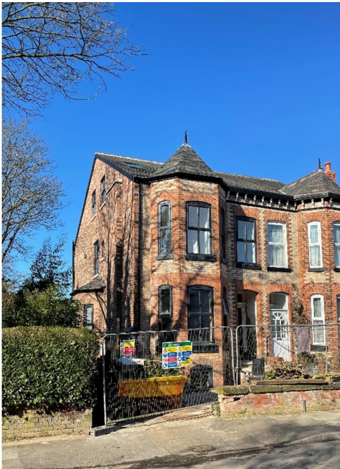
Front elevation of 8 Brunswick Road,
