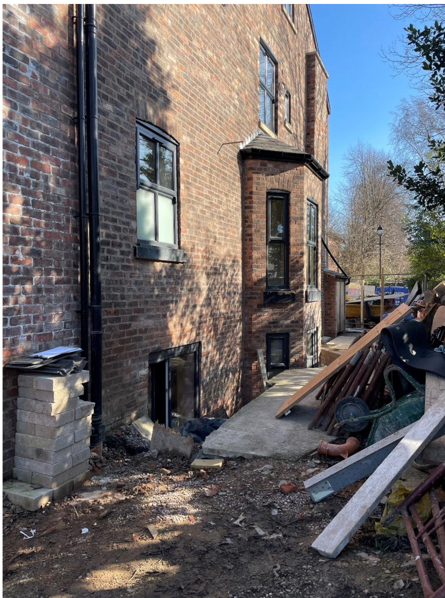
View of side lightwell and meter housing from rear
