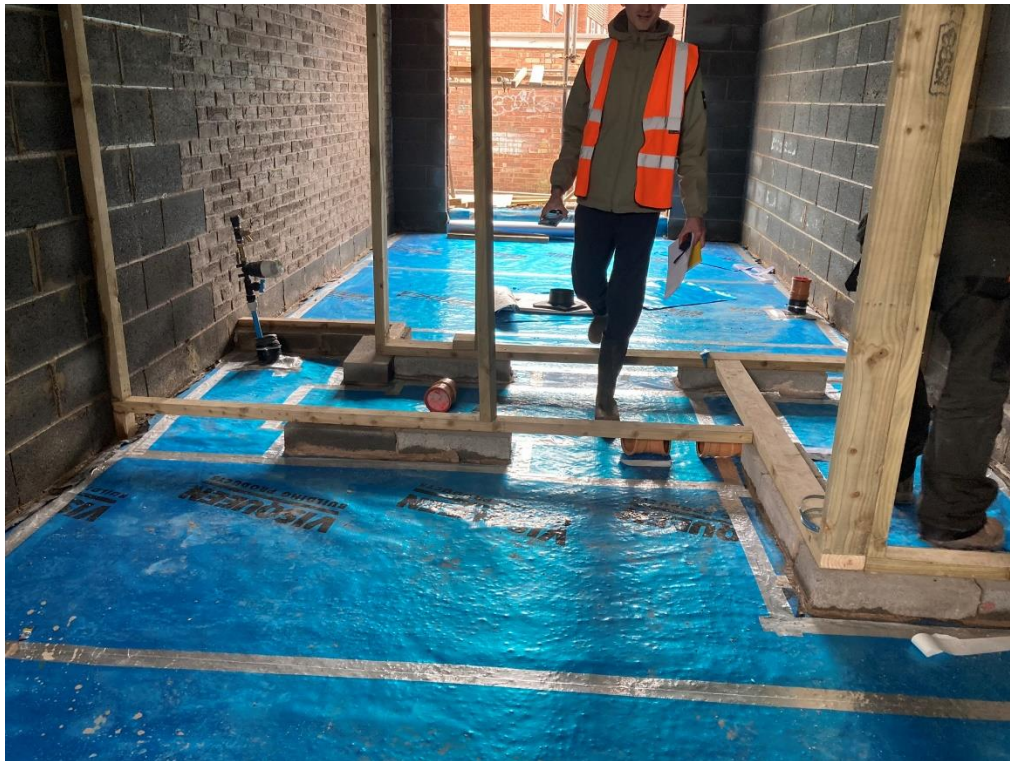
Photograph 11: Overview of Plot 2 (October 2020).
