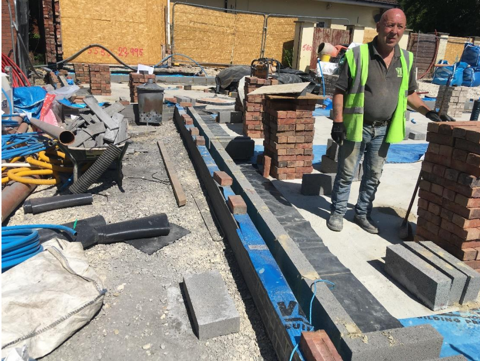
Photograph 1: Plot 1 perimeter membrane and DPC installation (May 2020).
