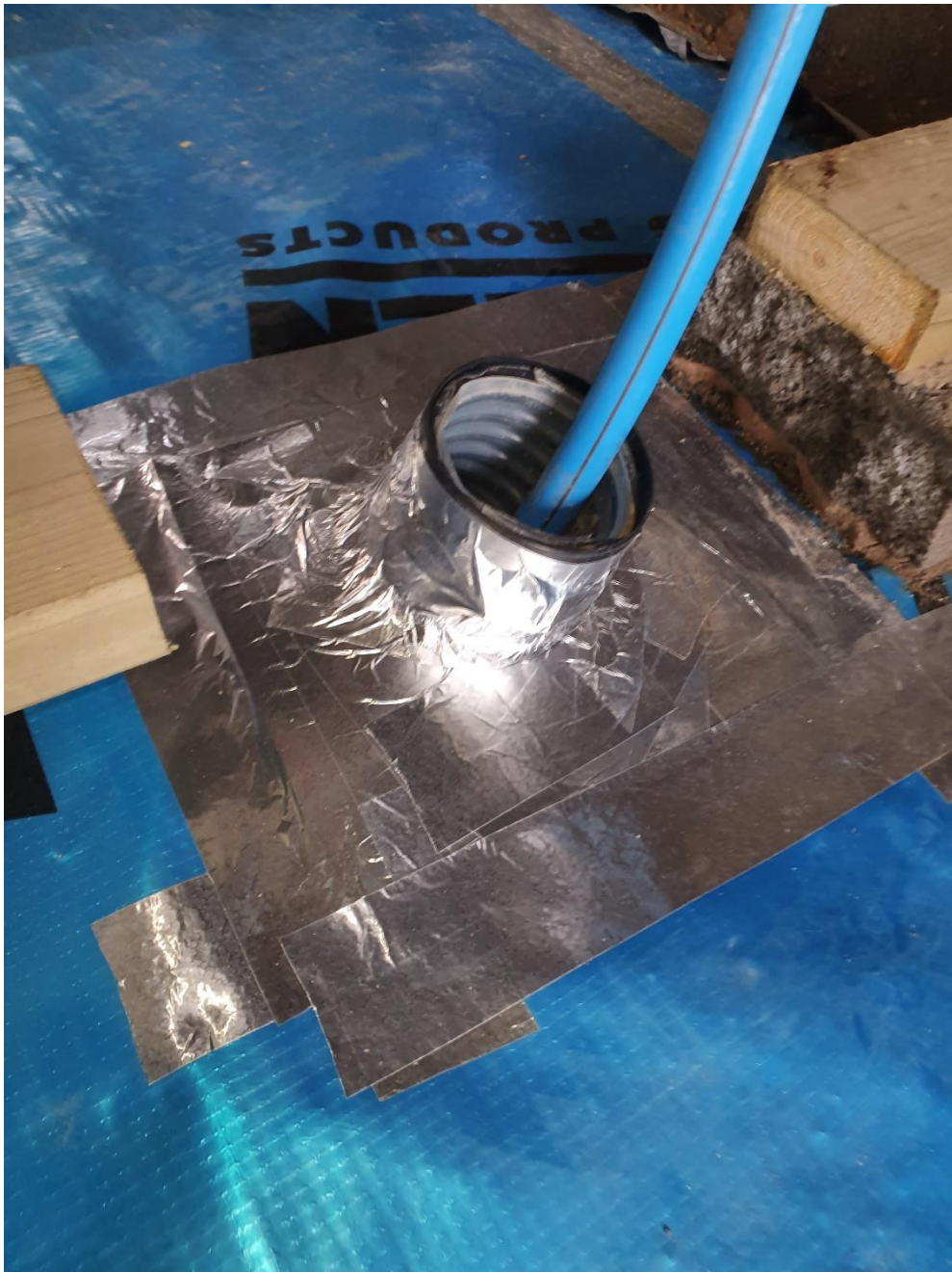
Photograph 6: Tidying / repair of area shown in Plot 3 in Photograph 5 following EDGE inspection (October 2020).
