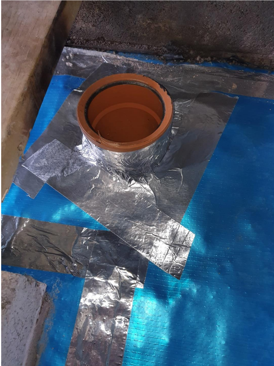
Photograph 10: Repairs to area shown in Photograph 9 (October 2020).
