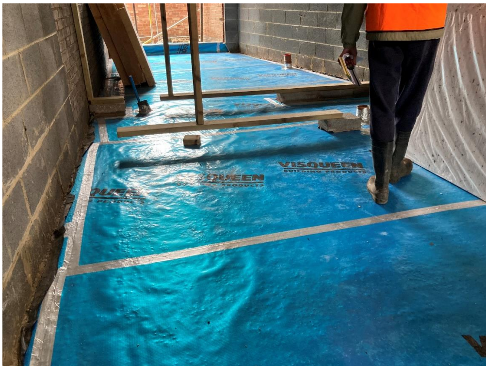
Photograph 12: Overview of Plot 3 (October 2020).
