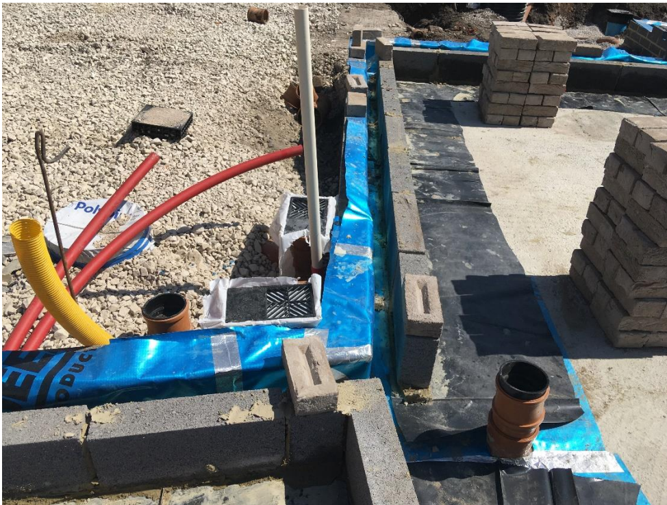
Photograph 2: Corner of Plots 3 & 4 showing membrane perimeter and DPC spanning cavity (May 2020).
