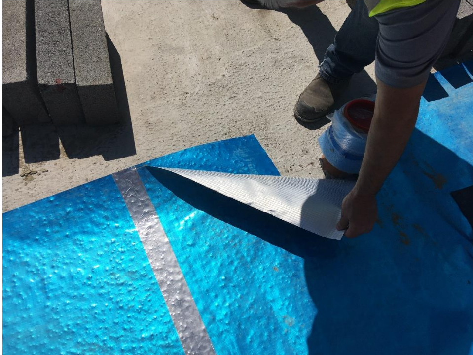
Photograph 3: Overlapping of membrane sections (May 2020).
