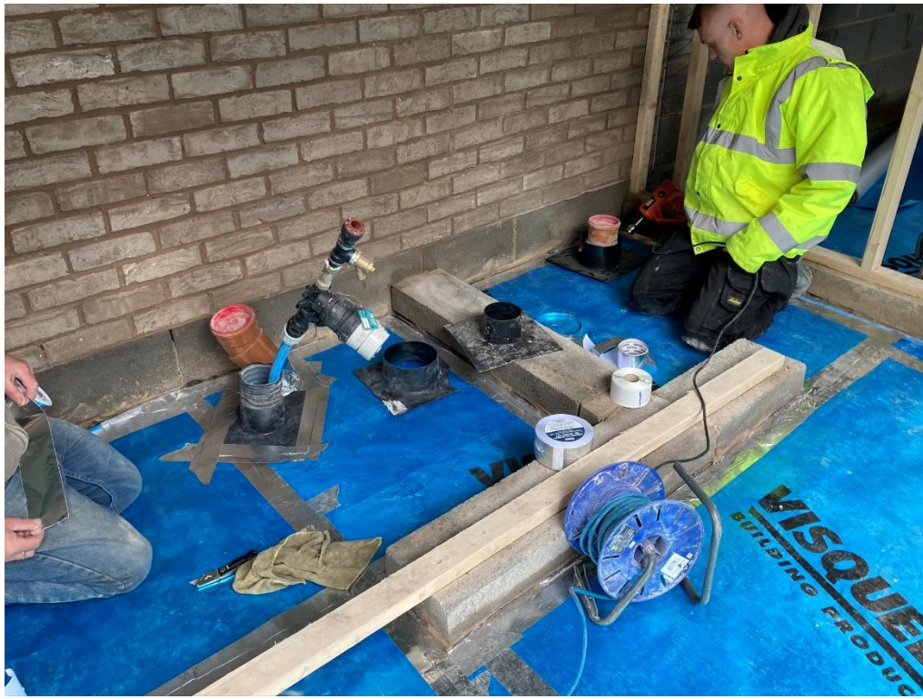
Photograph 13: Plot 4 membrane under construction.
