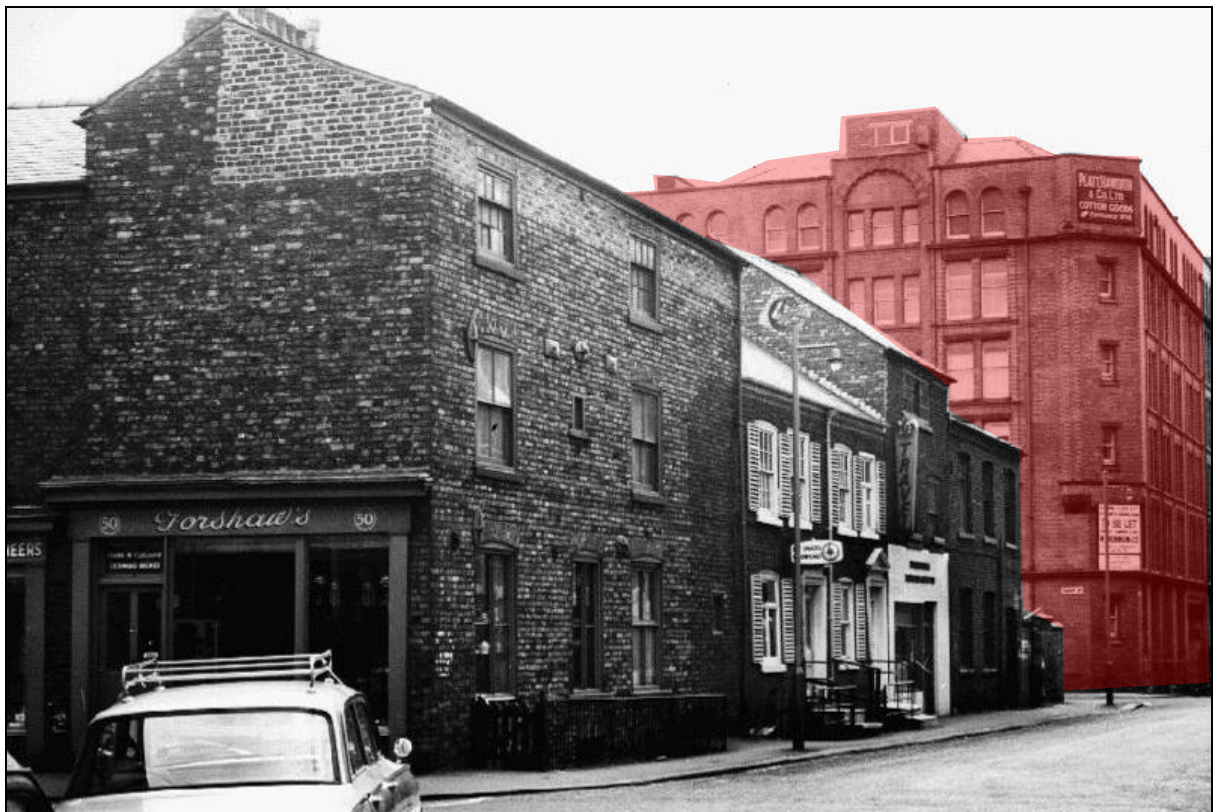
Figure 8: Looking east along Hilton Street in 1966, showing the exterior of Fourways House following the removal of the original decorated brick gables and chimney stacks at some point between 1960 and 1966. (Manchester City Archives).
