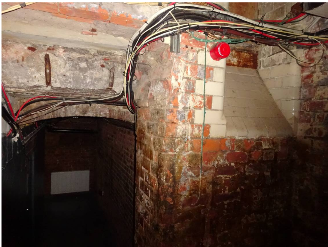
Figure 20: The bottom of the northern staircase, showing barrel-vaulted corridor beneath the loading bay (atrium reception) above. The glazed brick opening would have originally functioned as a vent or window to ground floor level.
