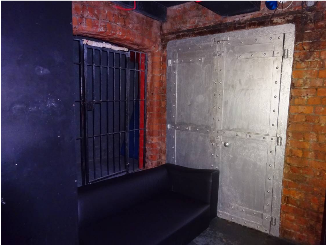
Figure 21: One of the original hoist doors and exposed brickwork.
