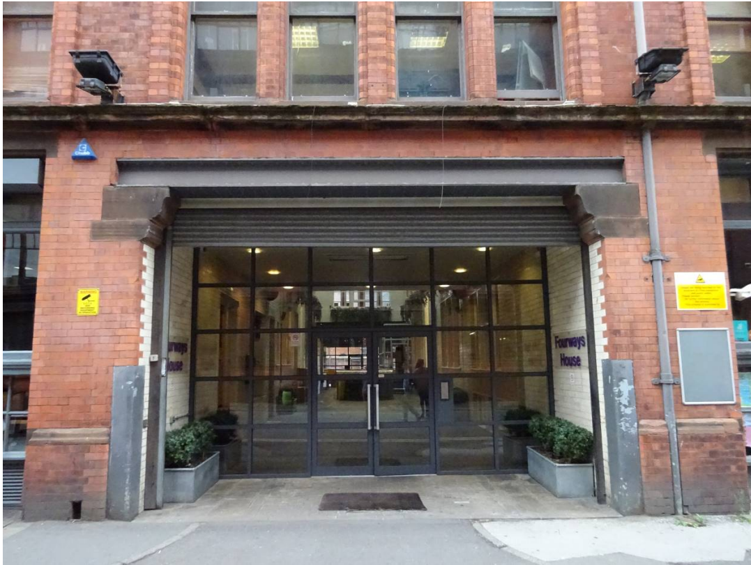
Figure 11: The original loading bay linking Hilton Street with Brewer Street to the east. This was converted into the main entrance into the building with the insertion of a glazed roof and external doors in 2001.
