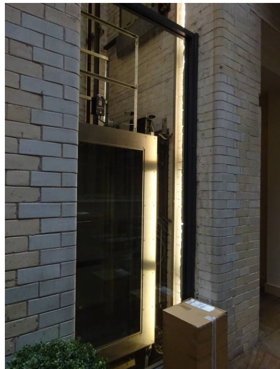
Figure 24: The modern lift located in the original hoist opening to the south of the space
