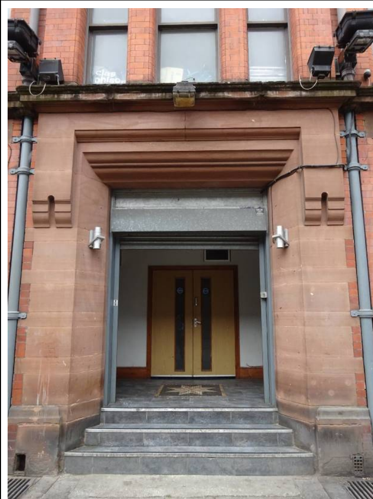
Figure 13: The entrance into No. 16 Tariff Street.
