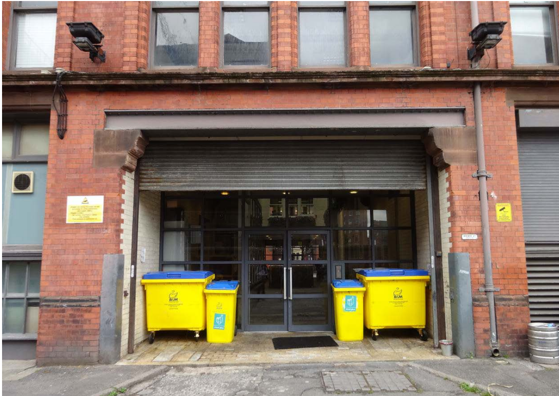
Figure 15: The rear of the original loading bay through the building as seen from Brewer Street.
