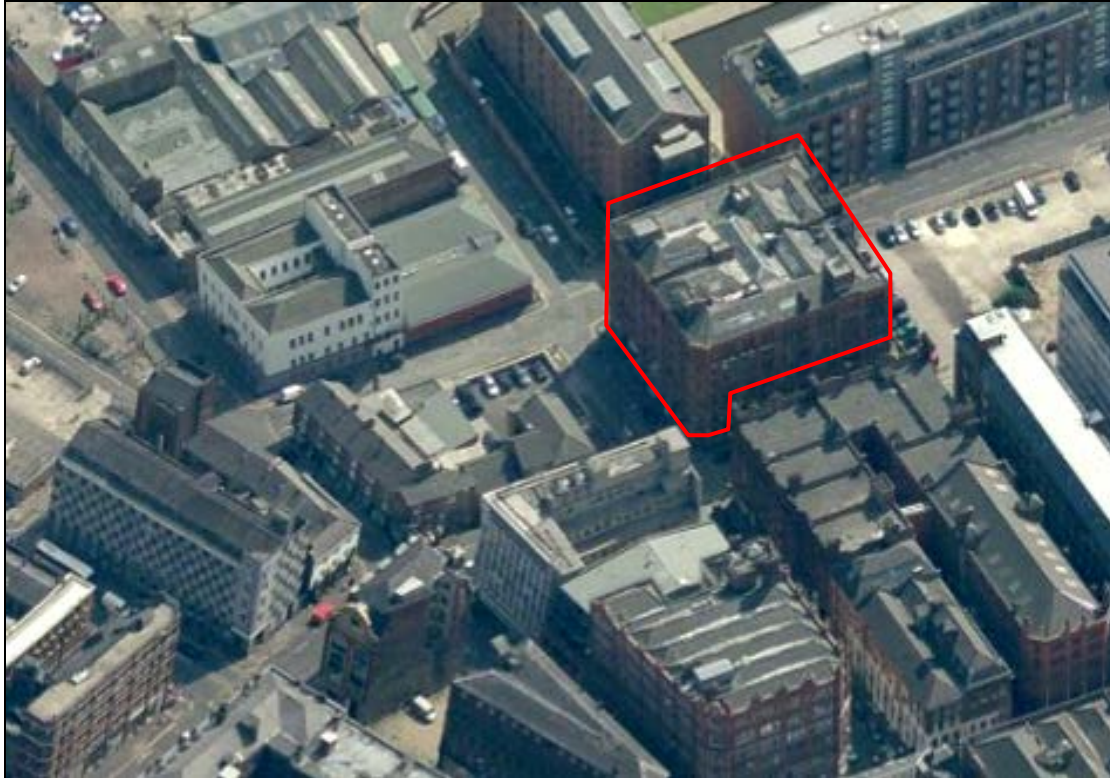
Figure 2: An aerial view looking north across the Subject Site (outlined red). (Manchester City Archives).
