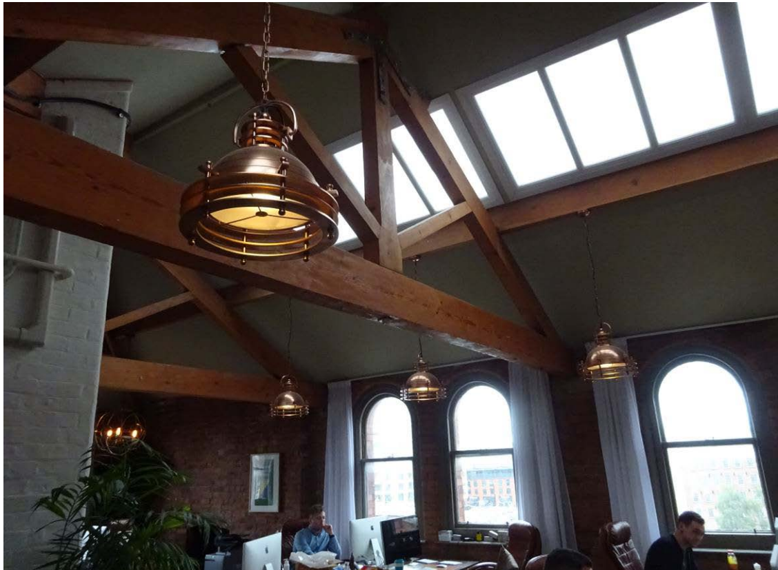
Figure 27: One of the office suites located within the top floor and roof space, showing the exposed original roof structure.
