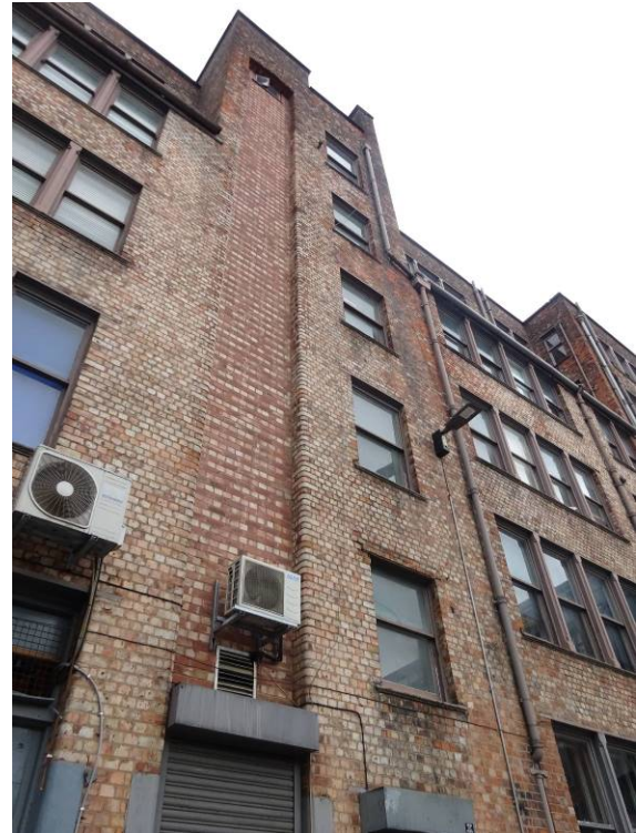
Figure 18: The now blocked external hoist.
