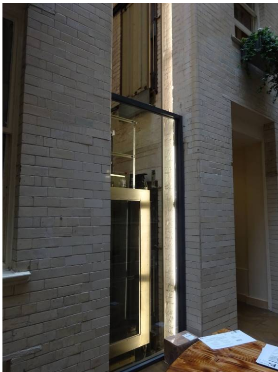
Figure 23: The modern lift located in the original hoist opening to the north of the space
