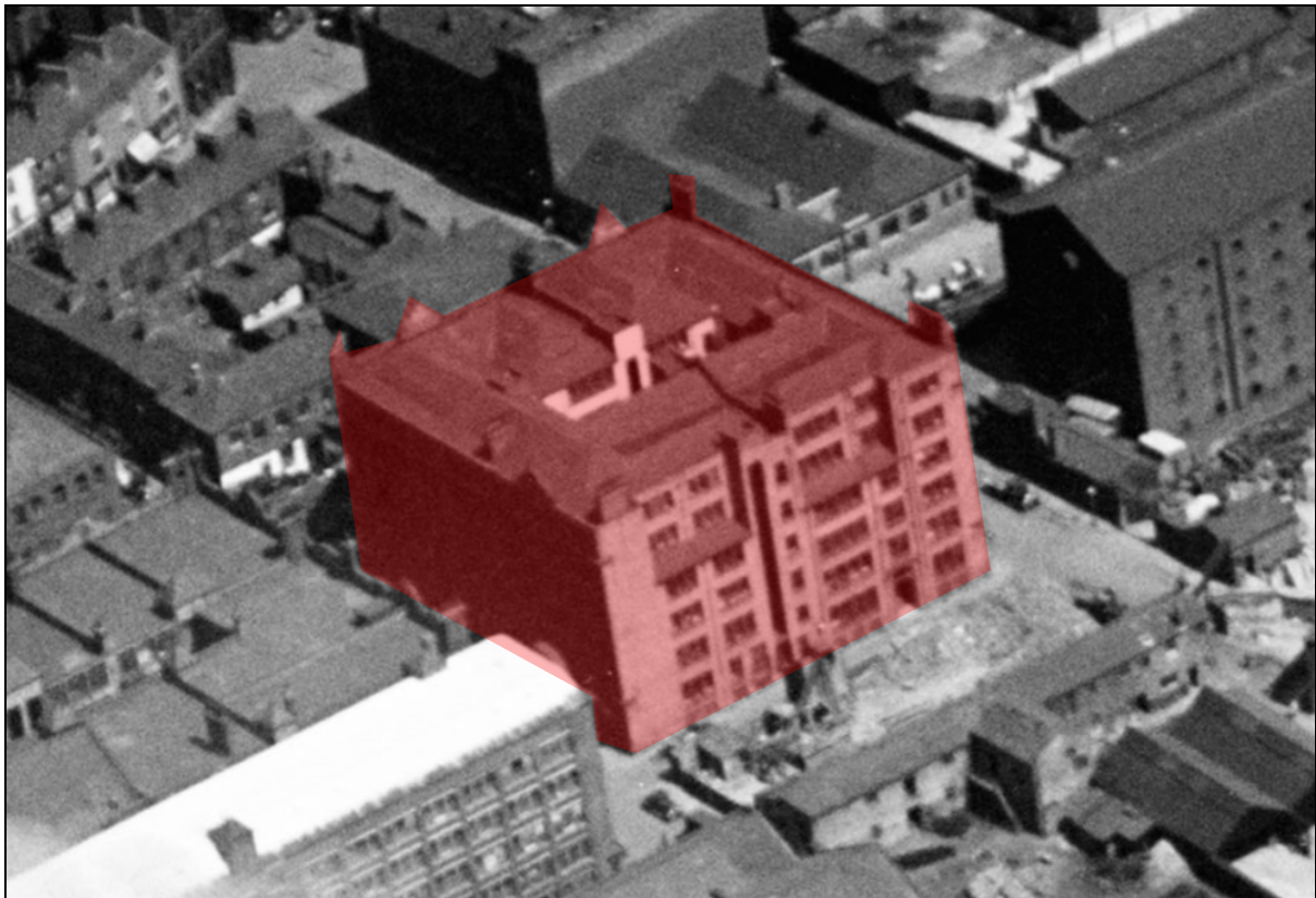
Figure 6: An aerial view looking north over Fourways House in 1932, showing the original chimney stacks and three gables defining the entrances into No.57 Hilton Street, and Nos. 16 and 18 Tariff Street. (Manchester City Archives).
