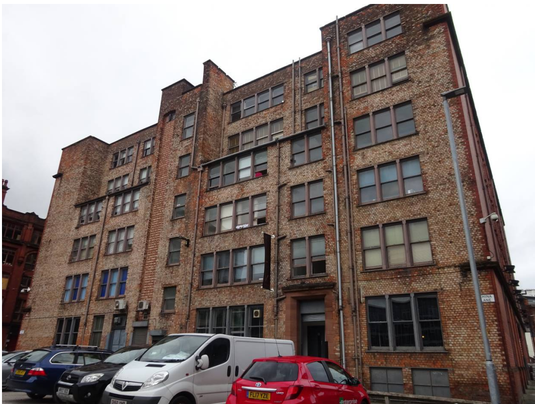
Figure 16: The south elevation on China Lane is entirely different in terms of design and materials. This elevation was located on a narrow rear street and was not afforded any unnecessary decoration or materials, and as such it uses cheaper Fletton bricks, asymmetrical fenestration, and the siting of an external hoist, now blocked to the left of the elevation.
