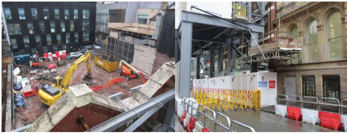
Figure 1; Photos showing the site (photo 1) taken from the south western corner and the remaining Invicta House façade along the southern boundary (photo 2)
