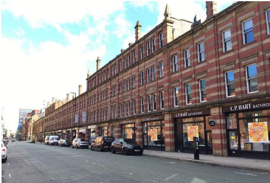
Figure 25 Former Entrance to Deansgate Goods Station including Nos. 223-233 Deansgate and 235-291 Deansgate as seen from the south-west
