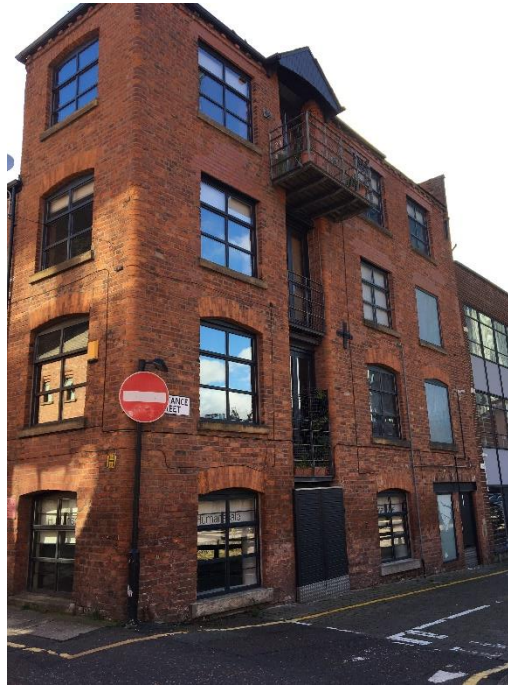
Figure 39 1 Constance Street/10a Little Peter Street as viewed from the north-west
