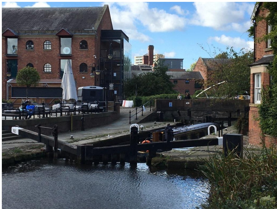
Figure 22 Rochdale Canal Lock No. 92 and Castle Street Bridge as seen from the east
