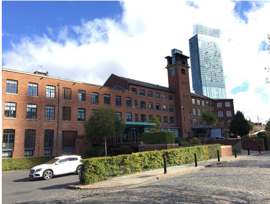
Figure 36 Eastgate (right) and Bass Warehouse as seen from the south-west
