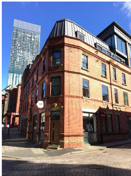
Figure 41 357-361 Deansgate viewed from the south
