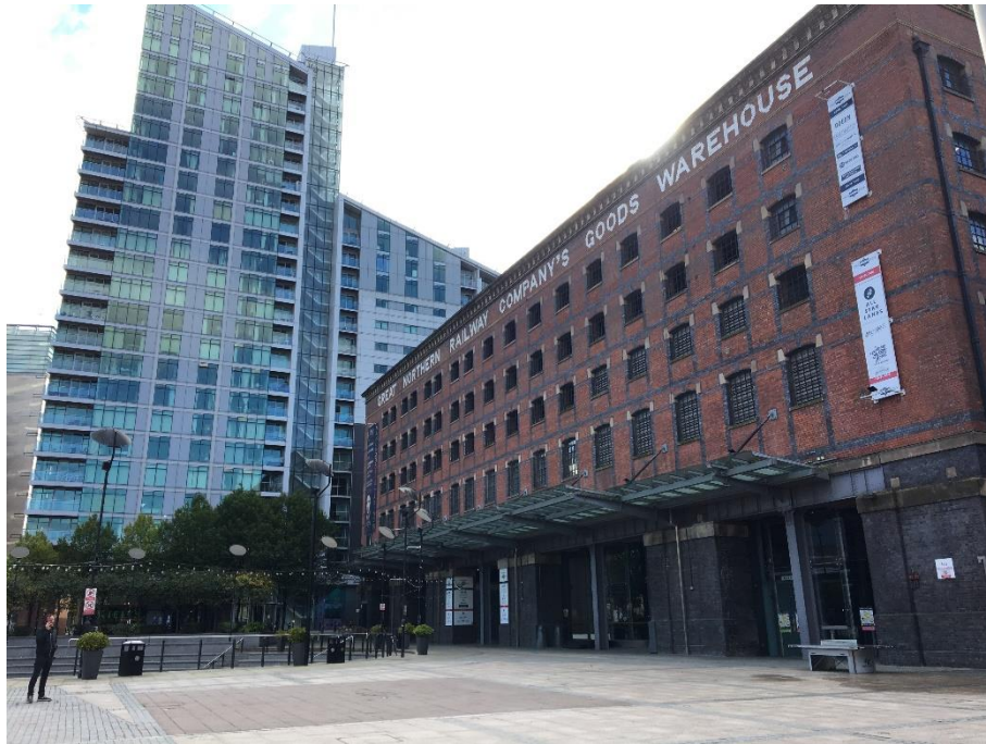
Figure 26 Deansgate Goods Station and Warehouse as seen from the north
