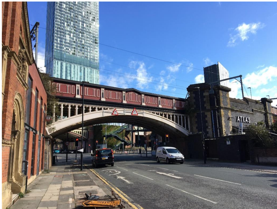
Figure 32 The Manchester South Junction and Altrincham Railway Viaduct viewed from the south on the Bridgewater Viaduct
