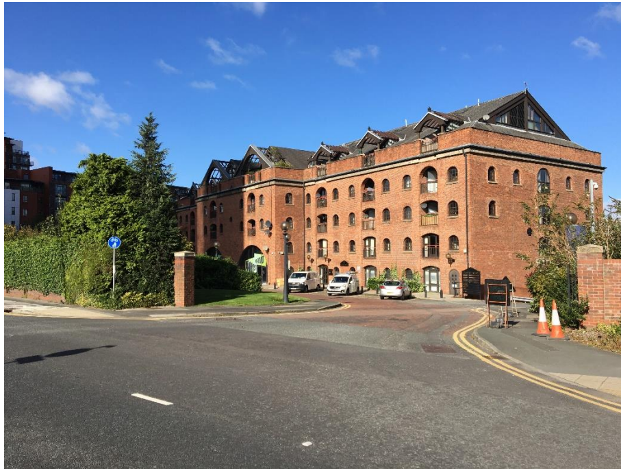
Figure 19 Middle Warehouse as seen from the south-east
