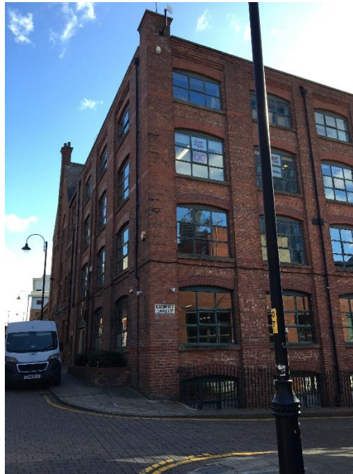
Figure 40 21 Little Peter Street/8-12 Hewitt Street as seen from the north-west
