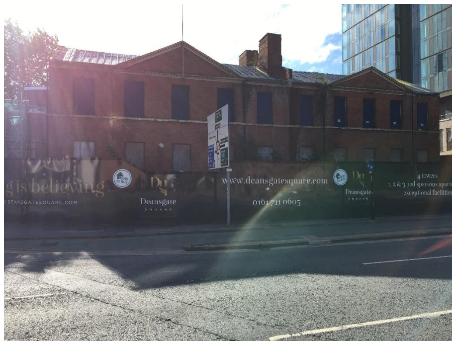
Figure 18 Bridgewater Canal Offices as seen from the north
