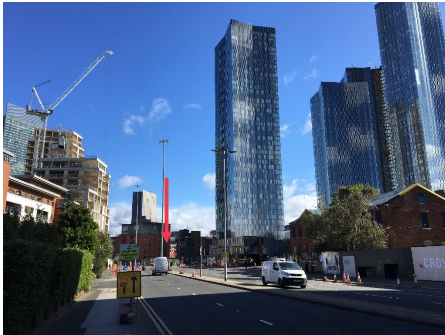
Figure 15 View looking east toward the site from the junction of Chester Road and the Castle Quay Access Road. The location of the site is marked by the red arrow
