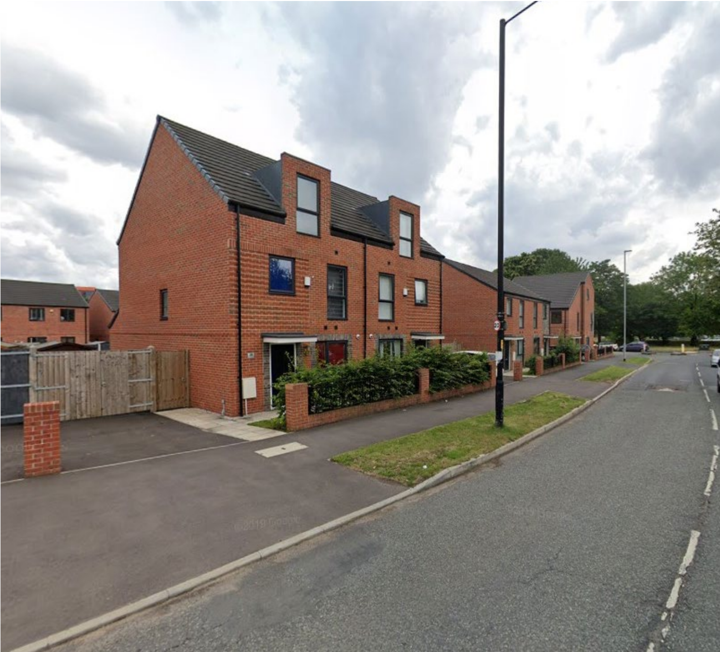
Housing located on Butler Street
