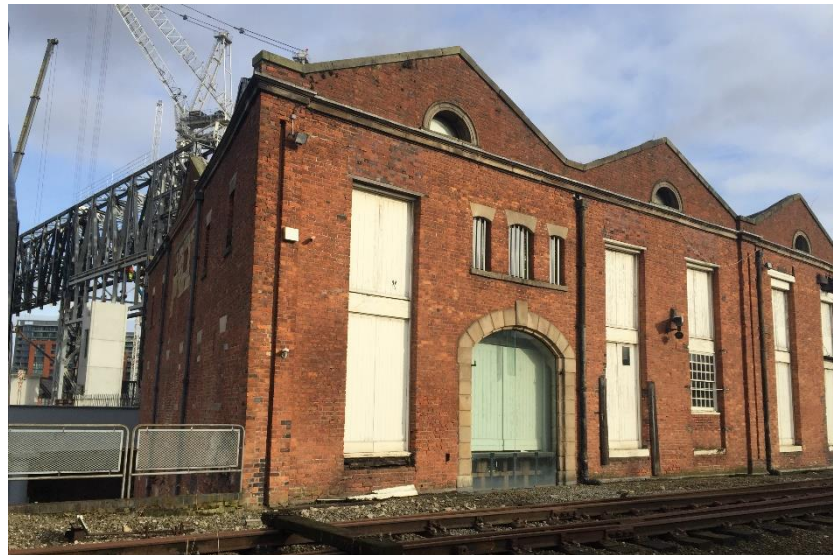
Figure 7: Bay 1, southern façade showing typical details.
