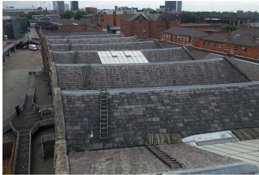
Figure 8: The roof today looking from Bay 1 to the east (Image from SDA).
