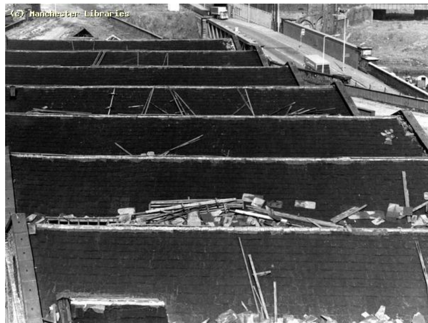
Figure 6: Photograph dated to 1978 showing the western end of the roof without skylights, bay1 in the distance to part of Bay 4 in the foreground (provided by SIMM).
