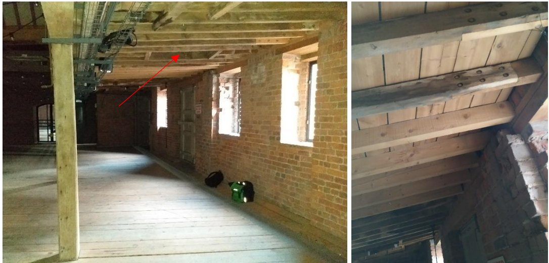
Figure 10: Bay 2, area beneath the mezzanine with existing hatch marked with an arrow and (right) example of typical restored mezzanine structure.
