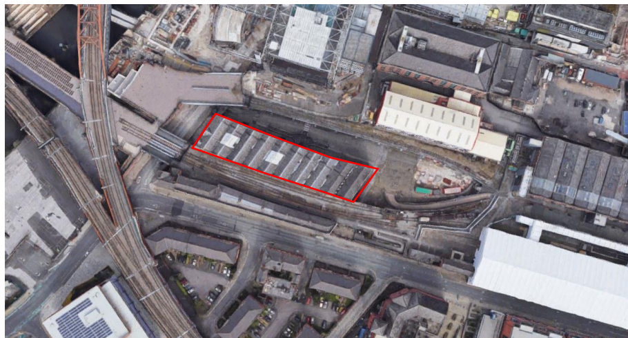
Figure 1: The 1830 Warehouse in context © Google Earth
