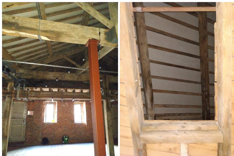
Figure 11 (left): slightly more distant view towards the Bay 2 mezzanine and area of the proposed hatch, note the existing hatch is concealed by the substantial beam on the front edge of the mezzanine.
