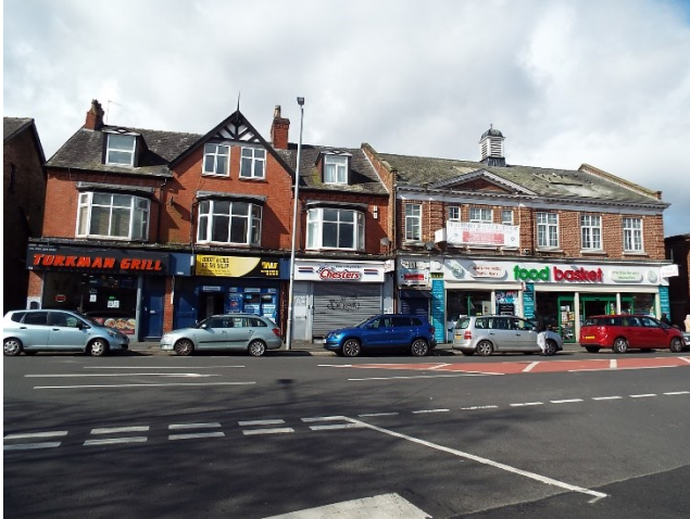
The west side of Withington Road
