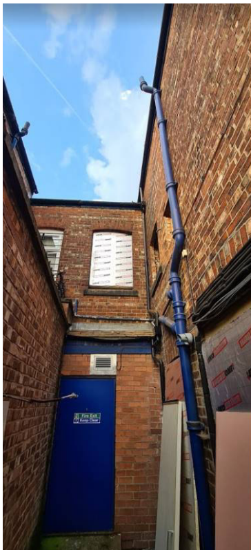
Courtyard towards Stockport Rd
