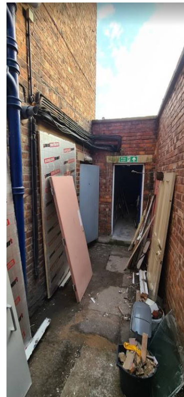
Courtyard towards Dencombe St
