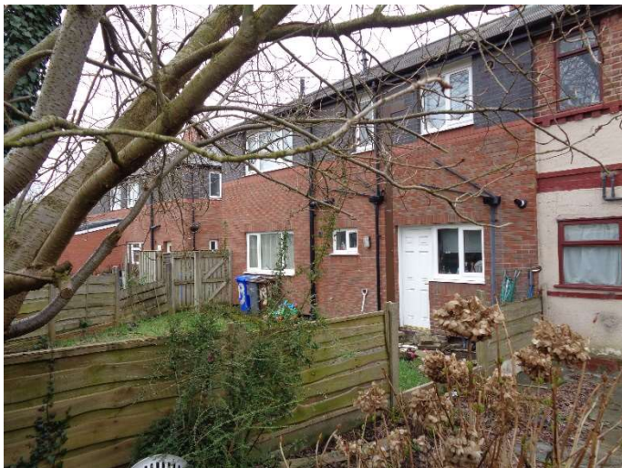
Rear Elevation towards 13/15 29 Longport Avenue
