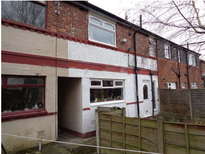
Rear Elevation towards 9 Longport Avenue
