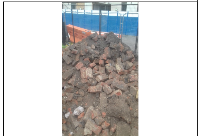
Trial Pit 101 Spoil
