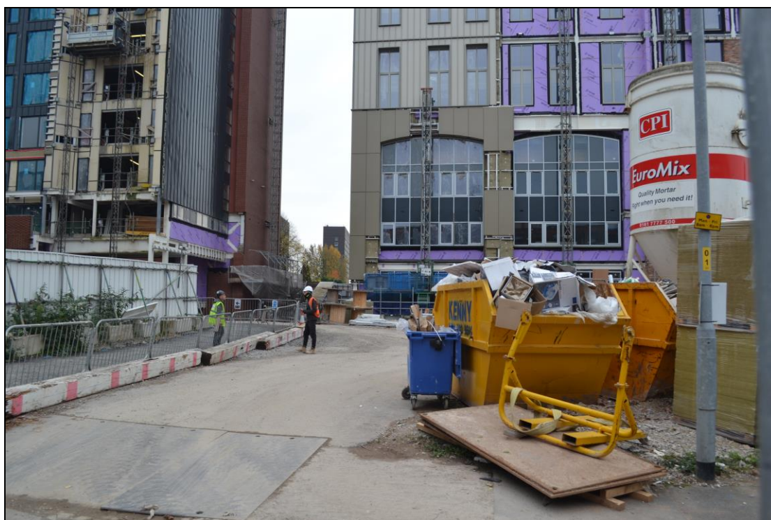
Photograph 7: View south within the PDA towards the Chester Road/Block C development.
