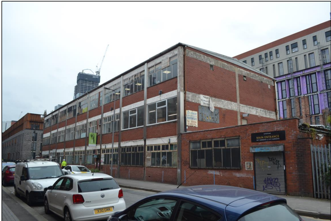
Photograph 1: View south-east of the northern and western façade of the former Phoenix Works.
