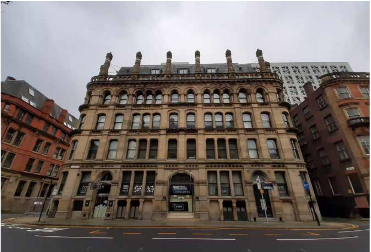
3.16 Princess Street principal facade
