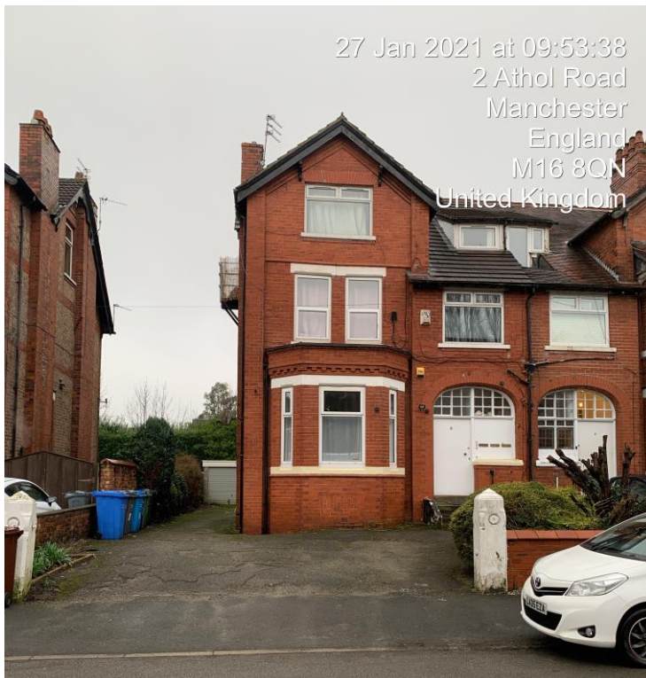
Photograph 1 Front Elevation as viewed from Athol Road
