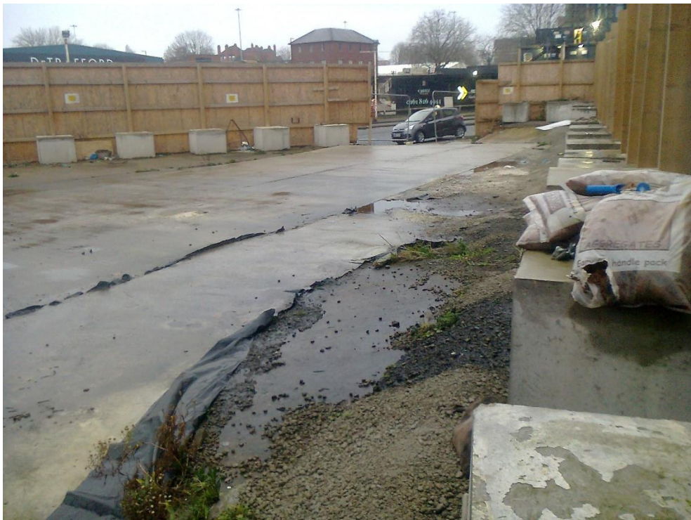
Photo 8: General site view looking south from northern corner
