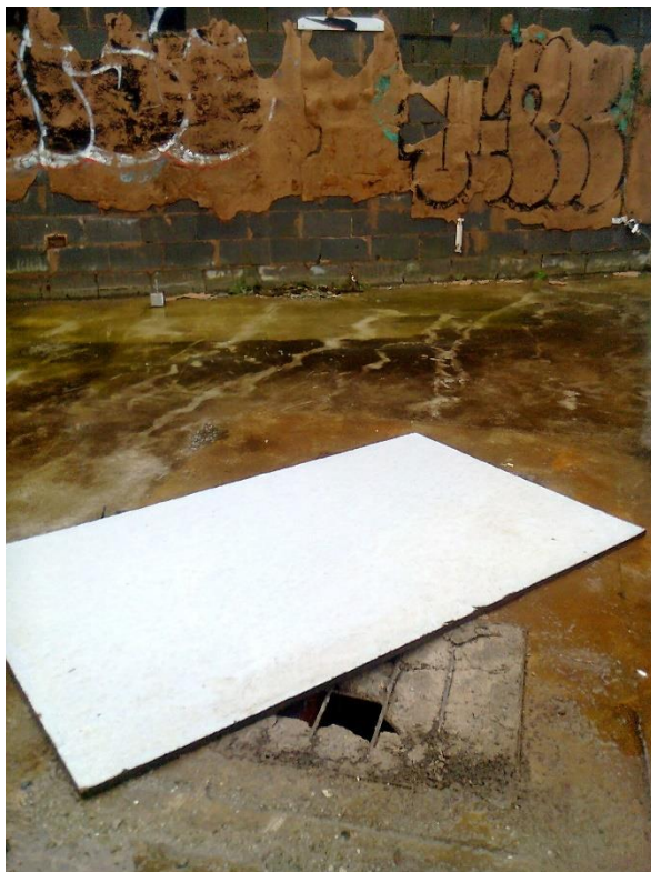
Photo 11: Broken manhole cover in eastern area
