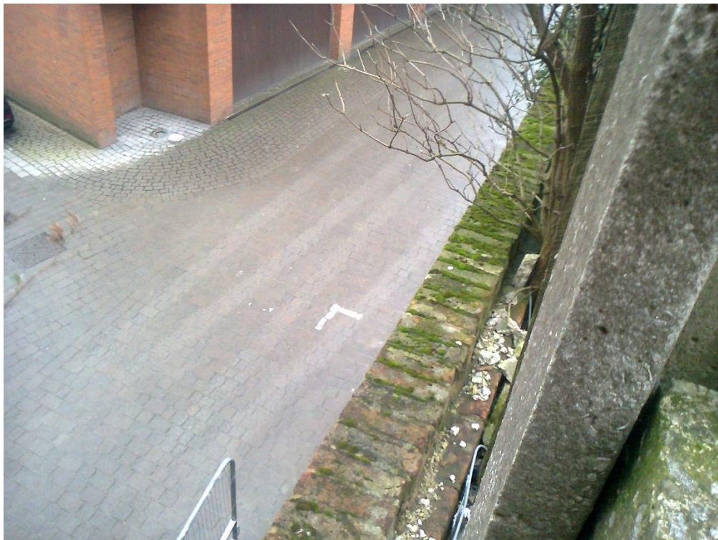
Photo 10: View down to access road beneath Bridgewater Viaduct, looking towards the southeast
