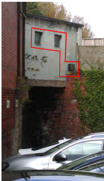
Opus photo 2015 – two windows and vent
