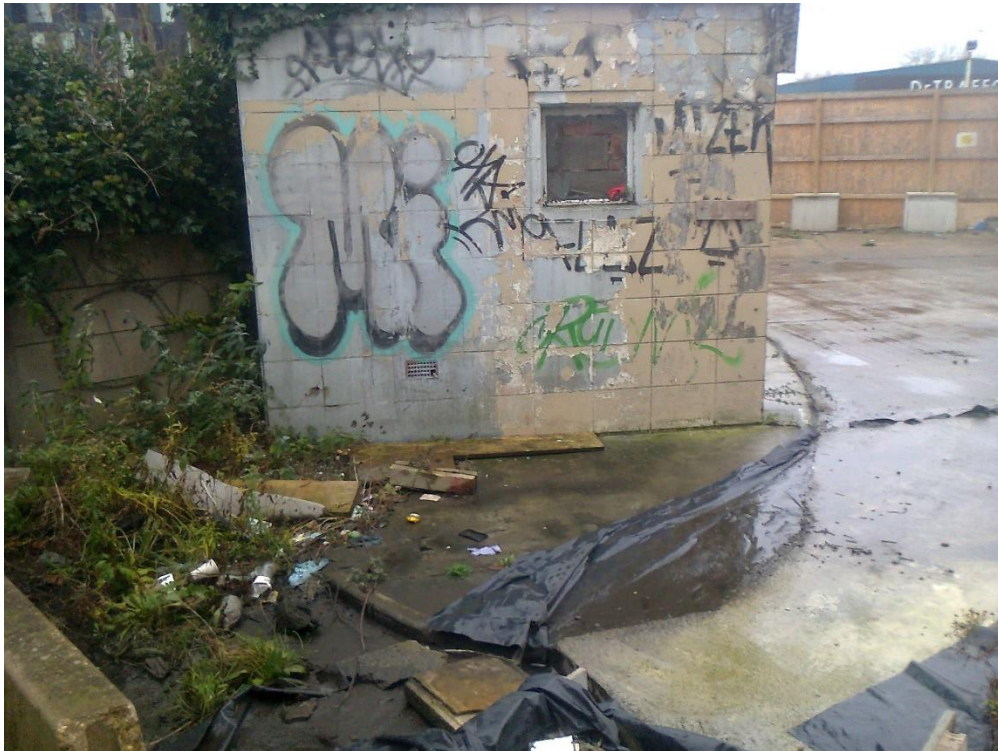
Photo 9: Northern corner showing west side of remaining wall
