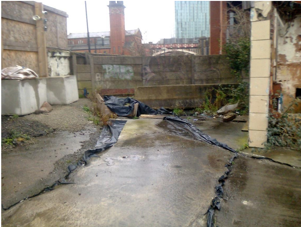
Photo 7: North western corner looking north
