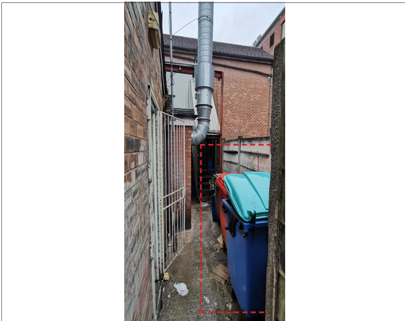
Fig 01 Image of the existing Industrial Bins located to the rear of the takeaway accessed via rear exit and from Grosvenor street.
