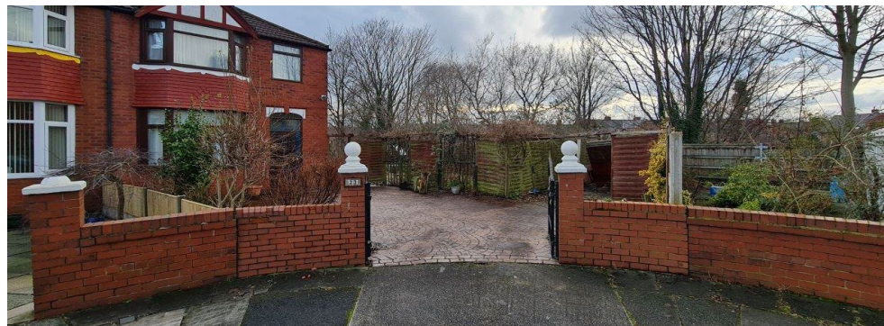
Front entrance boundary.
