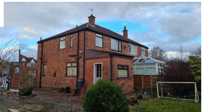
Photo of existing Garden area looking towards the Crimsworth Av
