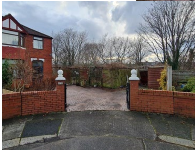
Crimsworth Avenue view of the entrance to the site
