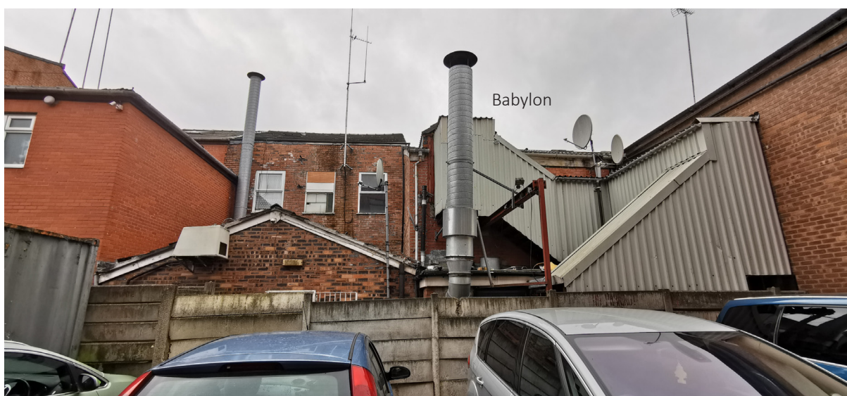
See Fig 02 Photograph showing the existing elevation of the rear of the building and the allocated area for air-conditioning.
