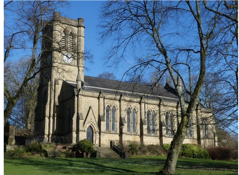
Figure 4.32: The tower and south aisle of St. Peter's Church
