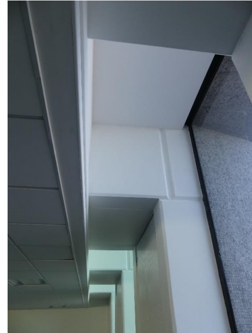
Figure 4.26: The modular structure adjoining the window openings of Floor 4
