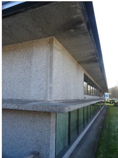
Figure 4.15: The deep reveal to the eaves and first floor canopy
