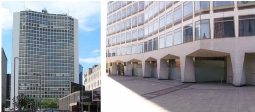
Figure 4.4: Alpha Tower, Birmingham (1972) (Seifert and Partners)
