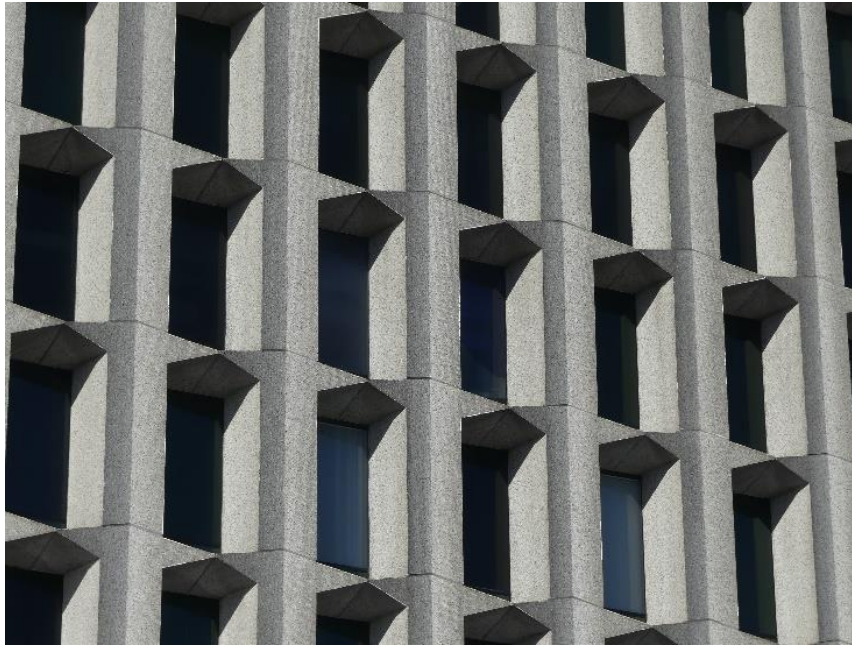
Figure 4.10: A detail of sculptural panels to the principal elevations
