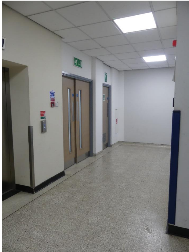
Figure 4.27: The lift lobby to Floor 9, original floor tiles remain, however the doors and ceiling have been renewed.
