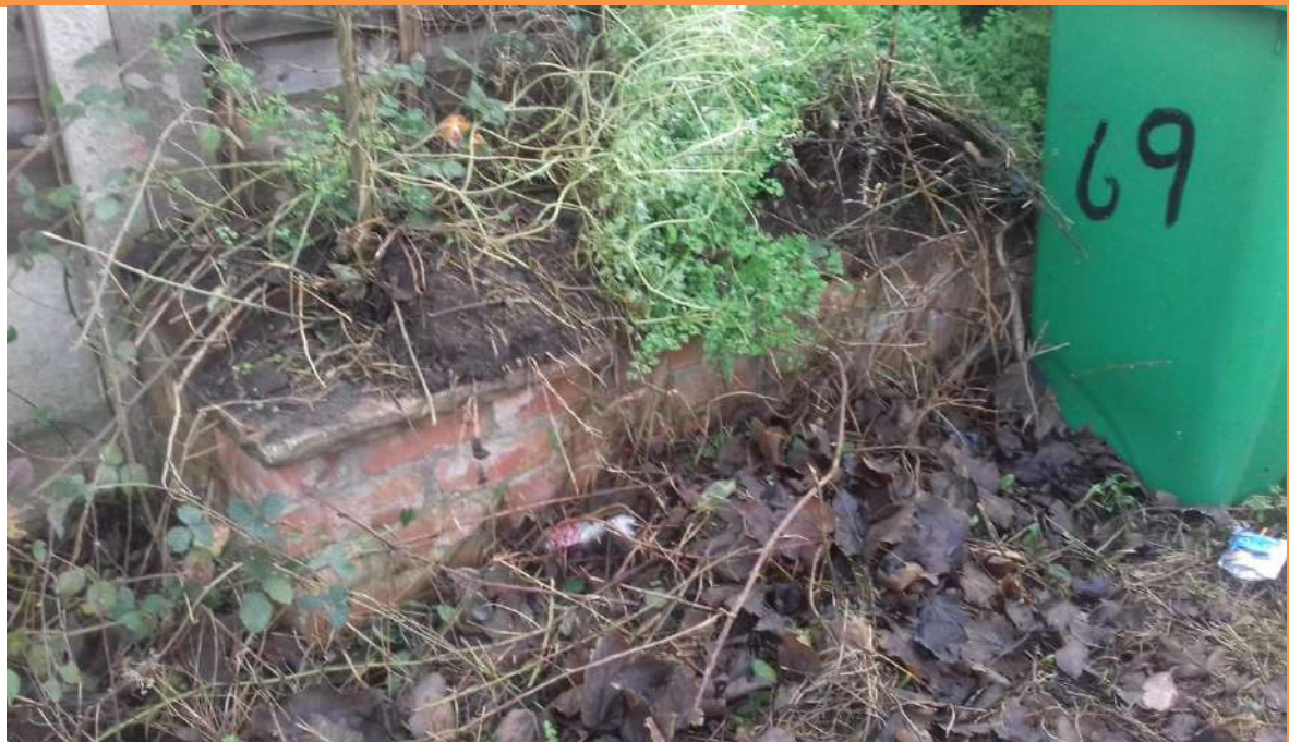
PLATE 10 – SMALL BRICK WALL ALONG EASTERN BOUNDARY
