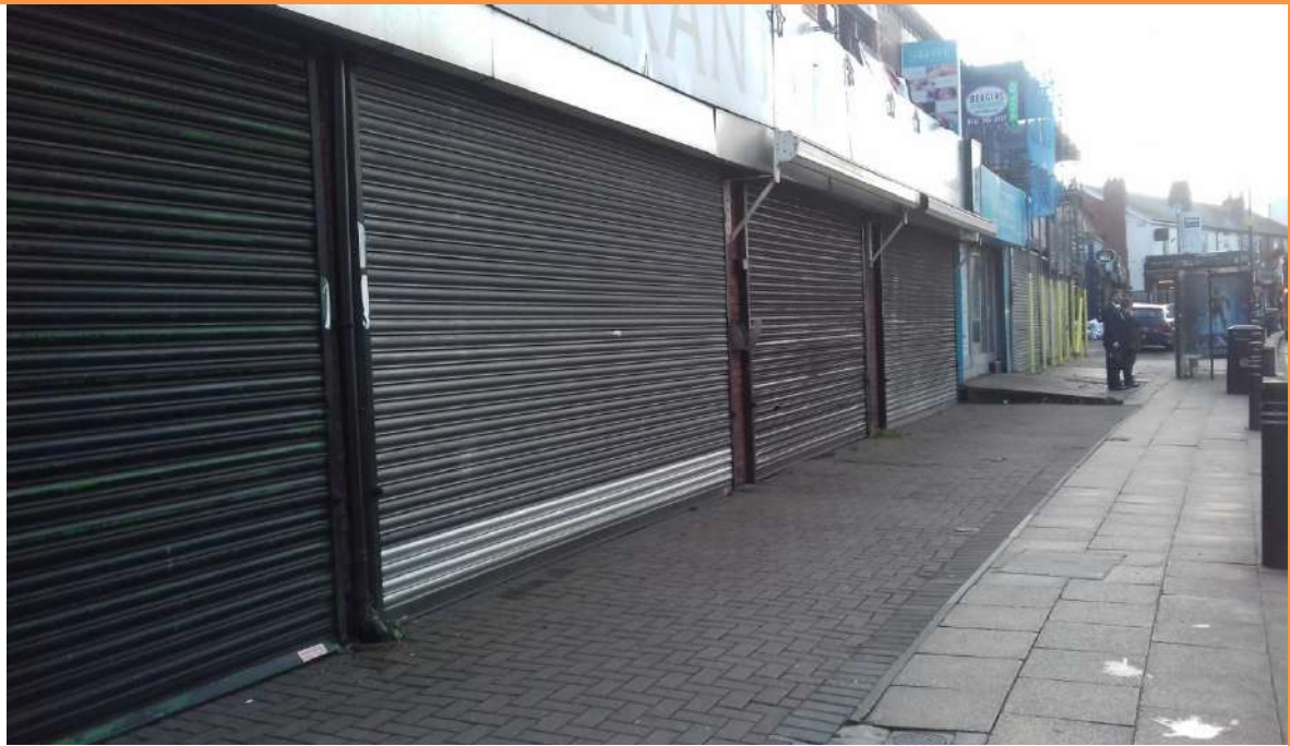
PLATE 1 – FRONT OF THE TERRACED BUILDING FROM PALATINE ROAD LOOKING SOUTH-WEST
