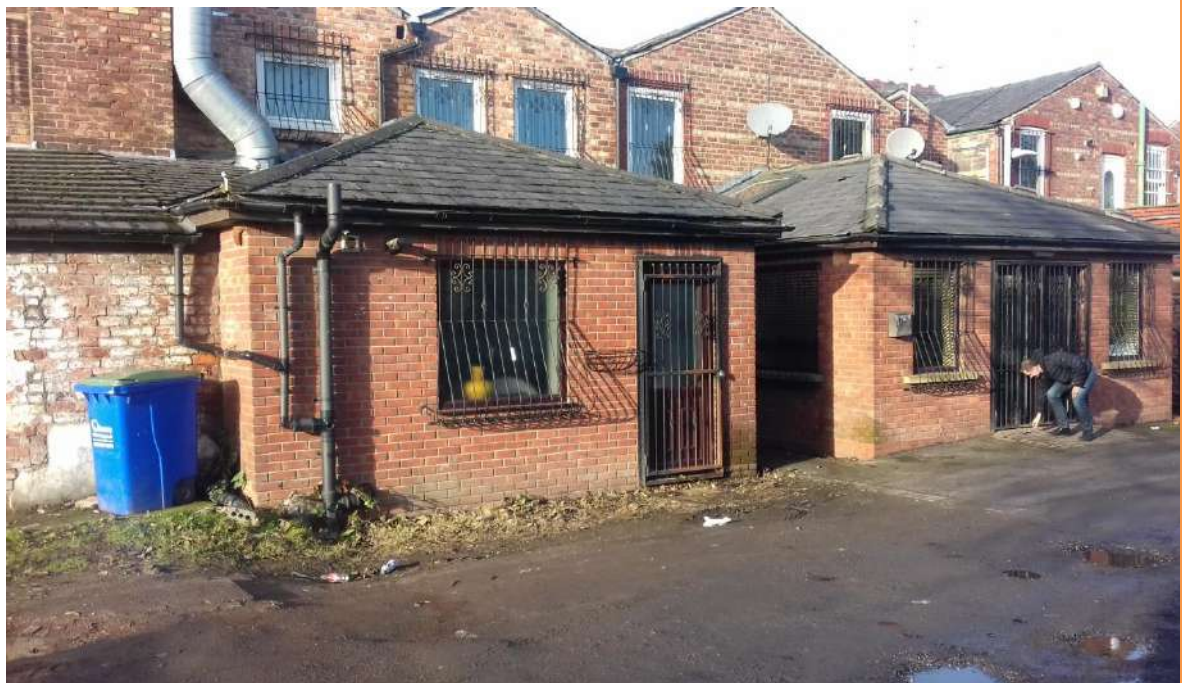
PLATE 6 – REAR OF THE TERRACED BUILDING LOOKING WEST
