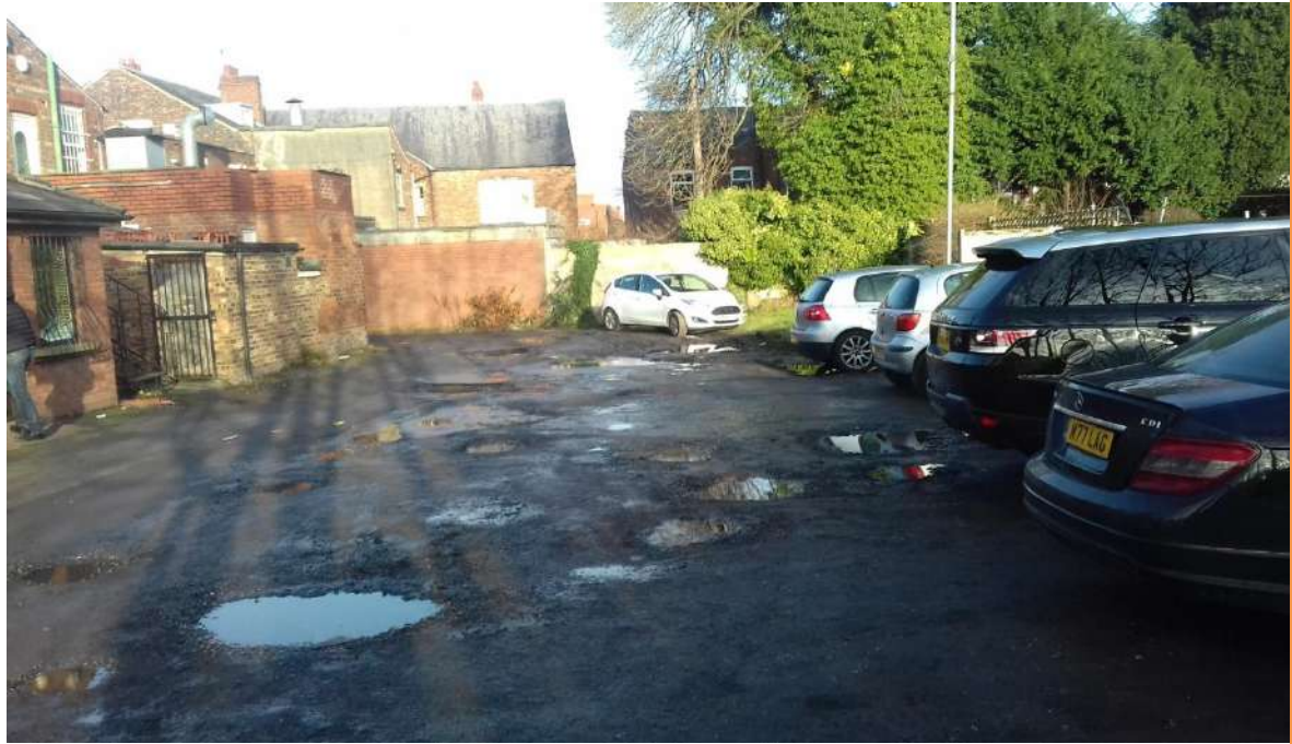
PLATE 5 – CAR PARK IN THE EASTERN SECTOR OF THE SITE LOOKING NORTH
