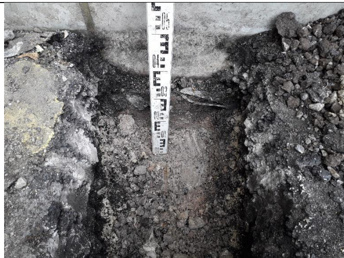
Trial Pit 01: Internal view of excavation
