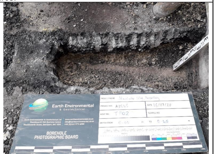
Trial Pit 02: Internal view of excavation
