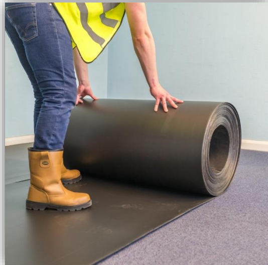
Floors - Protecta Board 1m wide (3mm)
