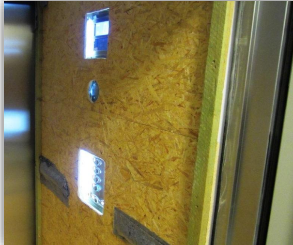
Example: Lift Protection with Ply board and pre-made cut-outs
