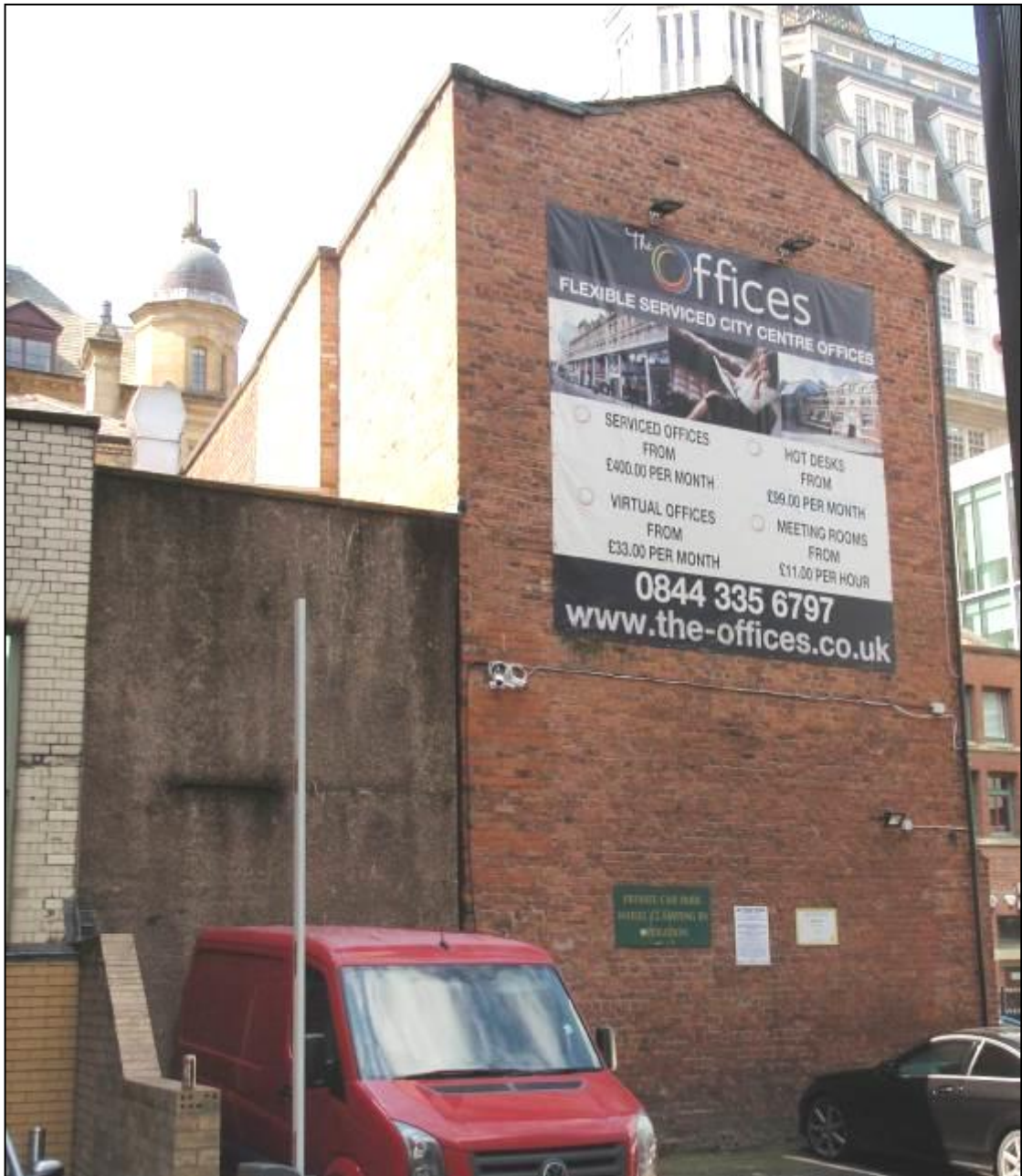
Fig 35: The mid-C20th altered rear outrigger adjoin the Magistrates' Court building.
