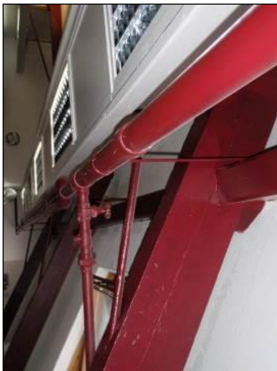
Exposed mid-C20th roof structure and lighting units – 2 nd floor all modern fittings of no significance.
