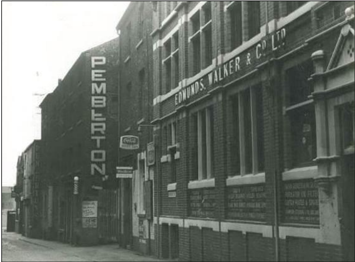
Fig. 26: Invicta House in 1968, looking west along Atkinson Street. The building was used as an office and car-parts warehouse for Edmunds, Walker & Co. Note the attached property on the west gable and the blocked basement lights. The former Hat Factory was located in the Pemberton Auction rooms, while the former J.H.Cuff Soda Works would have been located further east along Atkinson Street.
