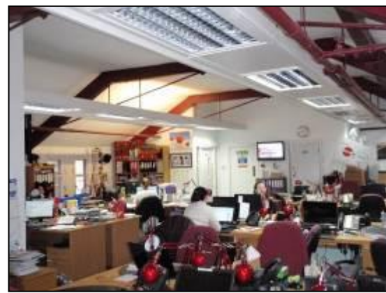
Open plan second floor office – mid-C20 roof trusses of no significance.
