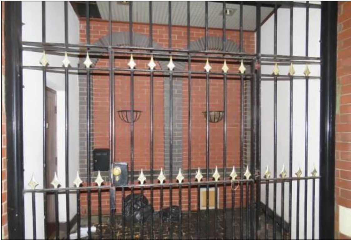
Fig 32: The infilled former carriage entrance to Atkinson Street.
