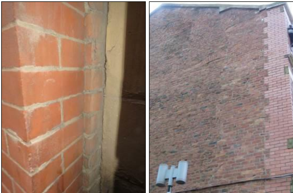
Fig 31: Details of the east and west gables of the façade, showing the abutment to the court house and the series of alterations to the Scott Place gable.
