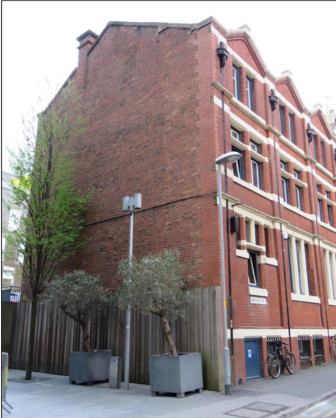
Fig 28: View east along Atkinson Street (April 2017) showing the 1900 façade. Note the number of blocked openings on the gable and the contrasting brickwork.
