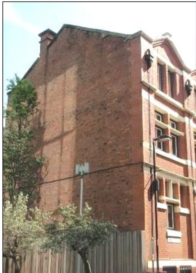
Fig 33: The exposed gable to Scott Place.
