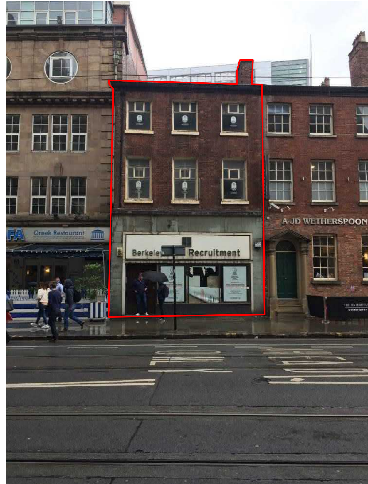
Figure 1 – Front elevation of 65 Princess Street
