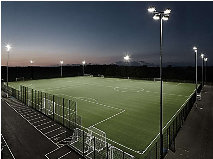
Typical 3G Artificial Grass Pitch (AGP) Installation
