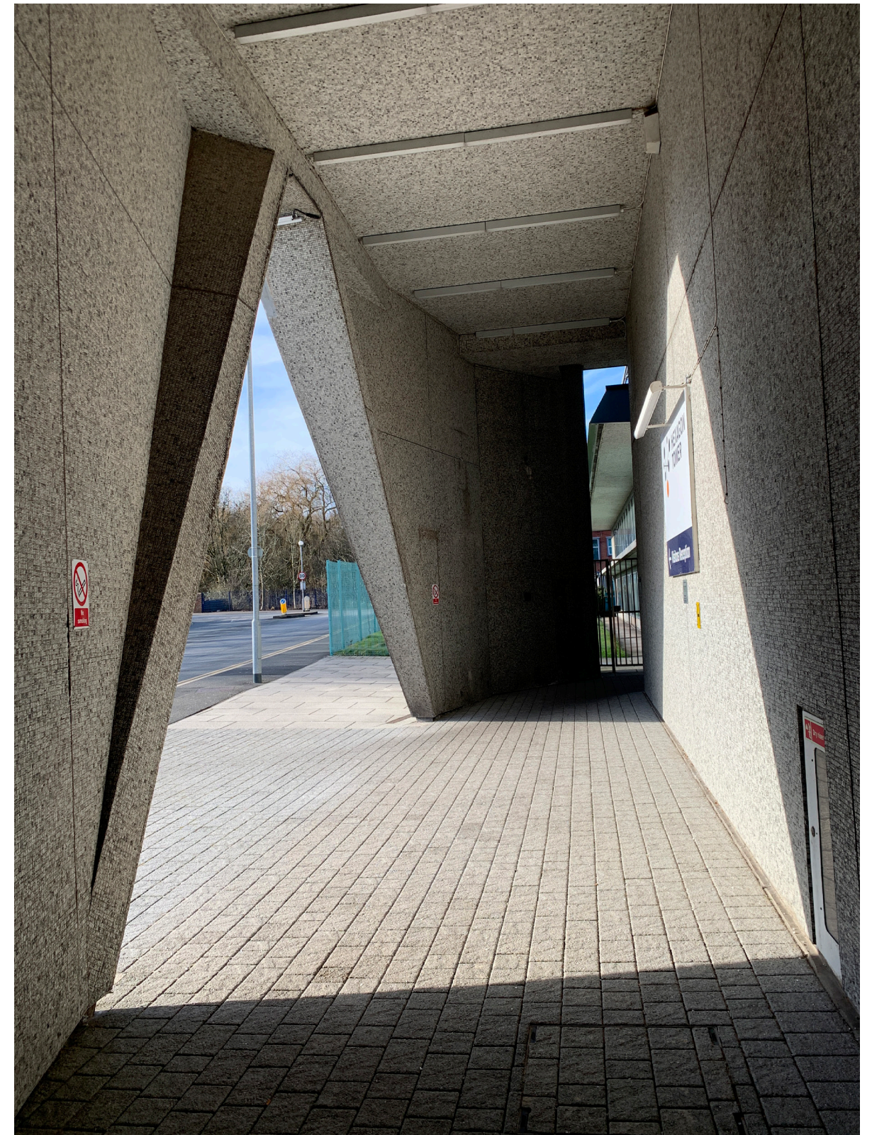
View of existing soffit at ground level to entrance on South elevation
