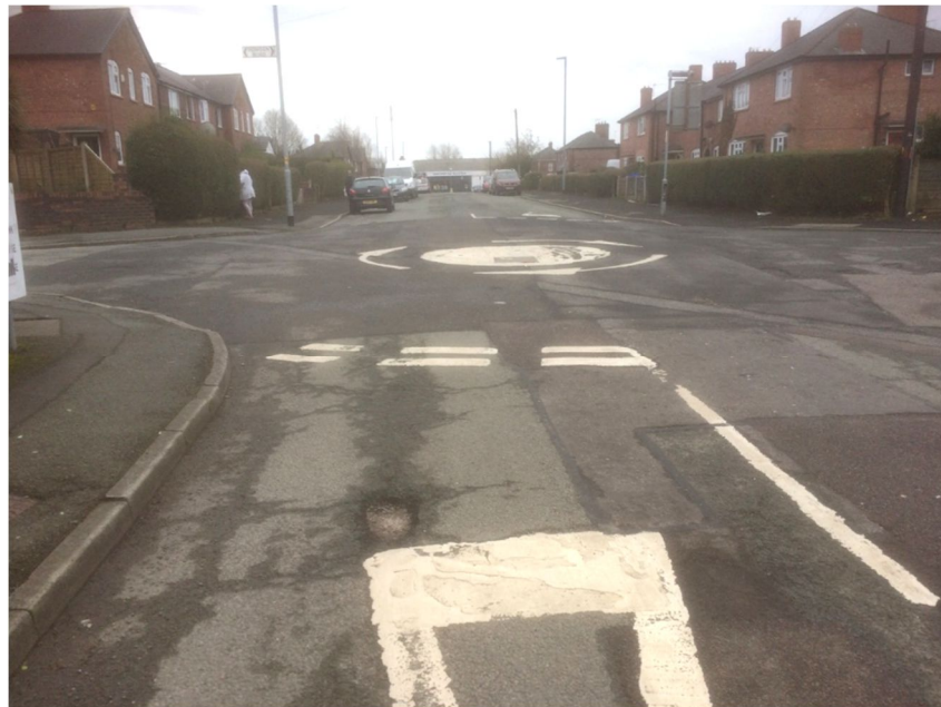
Figure 9: Junction of Boothroyden Road & Howden Road
