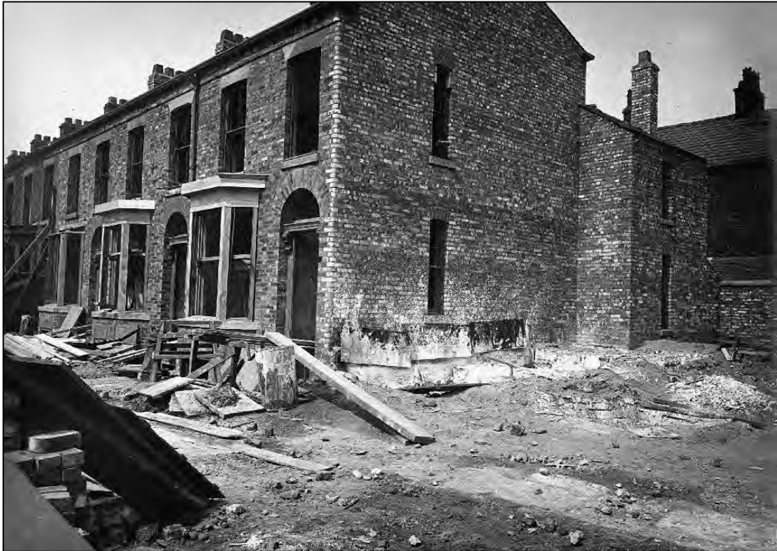
Plate 17: Halls Crescent, rebuilding of houses 1900
