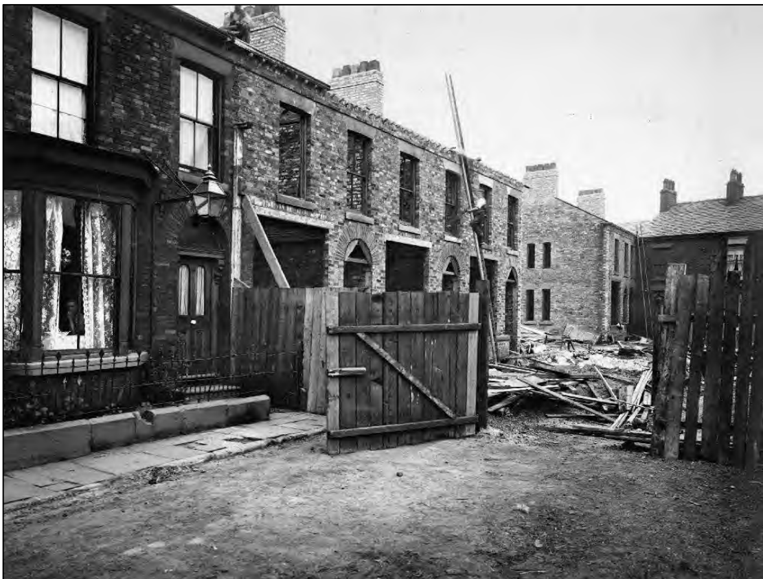
Plate 18: Hall's Crescent, near Rochdale Road, rebuilding of houses 1900
